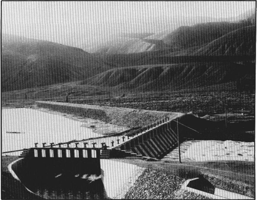
Derby Dam, completed by the reclamation service in 1905, diverted water from the Truckee River eastward by canal to the Carson River, thus decreasing the flow to Pyramid Lake. ( Nevada Historical Society )
