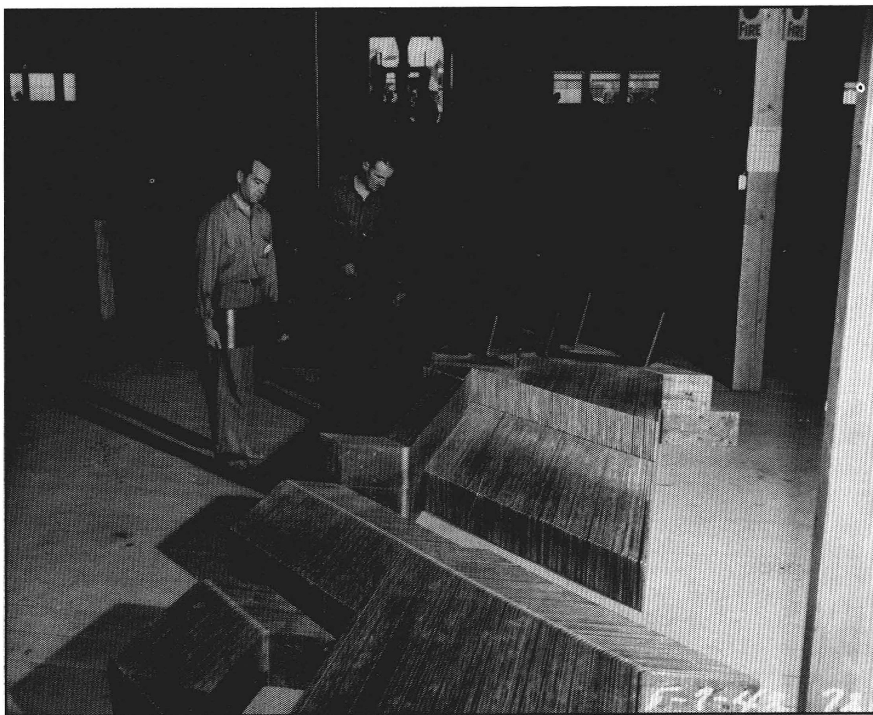
Stacking busbars ready for fill, BMI Plant, May 7, 1942. (Kunkel Collection, University of Nevada, Las Vegas Library)
