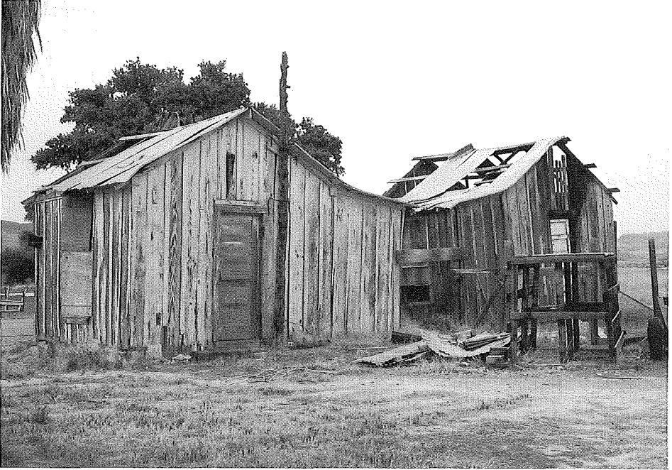
Former migrant worker dwellings on Liston Street in Overton in 1989. Some structures still remain as decaying reminders of the once booming farming industry in Moapa Valley. ( Corinne Escobar )
