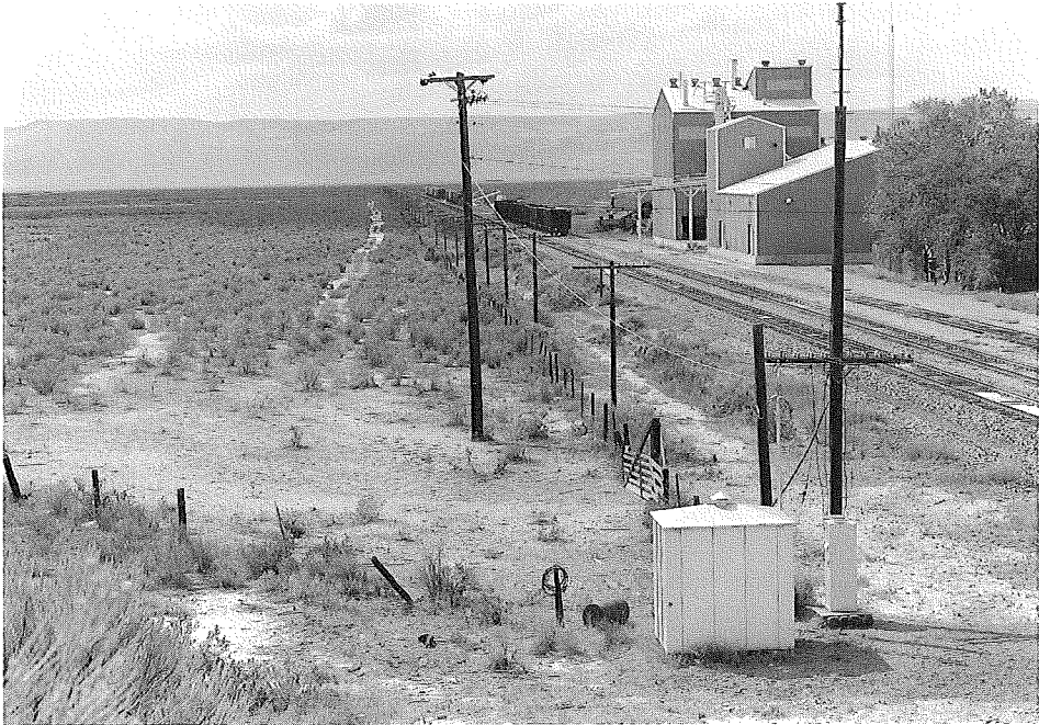
Dunphy Siding, Nevada, looking west
