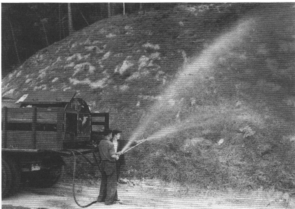
Hardis sprayer used for watering planted slopes on Wawona Road. Two men apply 3,000 to 3,500 gallons of water each evening after 5:00PM. (Note the two types of spray—one fine spray and one strong spray). (Collection courtesy of Yosemite National Park Library, Yosemite, California)
