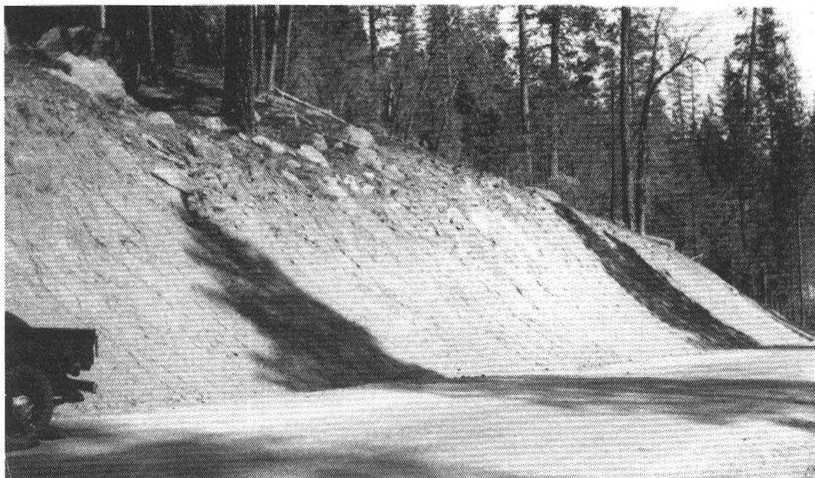
Wawona Road bank sloping—after picture, May 1936. (Collection courtesy of Yosemite National Park Library, Yosemite, California)
