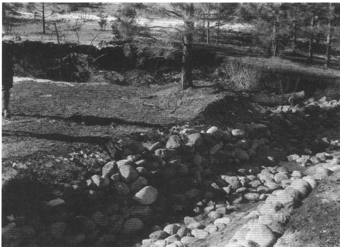
Deep gulley out in Wawona Meadow by uncontrolled stream. Shows new drainage ditch before gulley was filled, February 1936. Civilian Conservation Corps (CCC). (Collection courtesy of Yosemite National Park Library, Yosemite, California)
