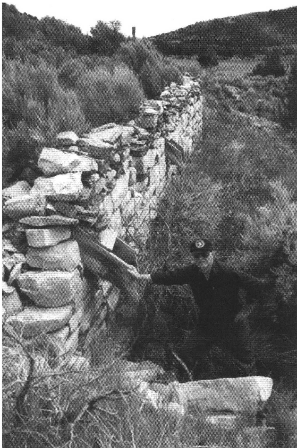
The feed chutes from the ore blending floor to the Stevenson Pans. ( Collection of the Author )
