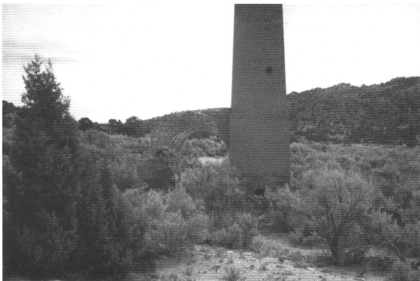
The Stetefeldt furnace at Belmont, Nevada, showing irregularity in brick construction. View toward the southeast. ( Collection of the Author )
