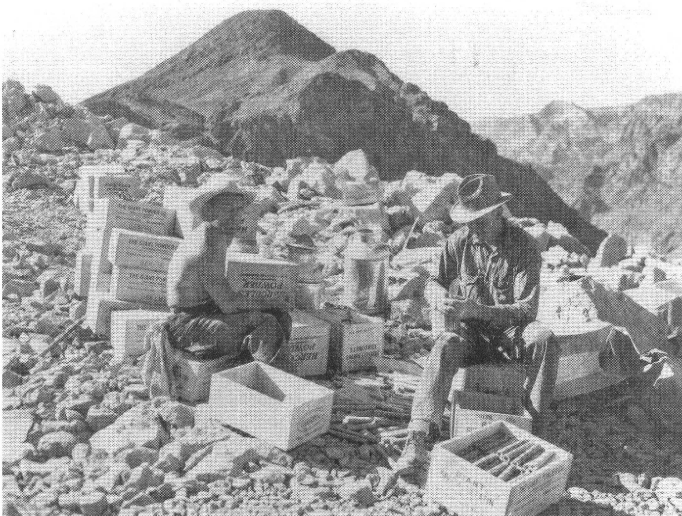
"Powder monkeys" loading dynamite sticks with electric primers, August 15, 1932. Photographer unknown. ( Boulder City Museum and Historical Association, McBride Collection )
