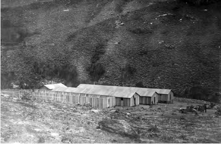
Camp Lamoille Barracks under Construction, 1933. ( Northeastern Nevada Museum Archives, Elko, Nevada )
