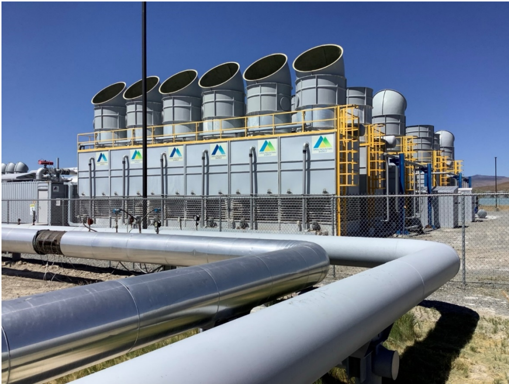
Figure 9. Cooling towers of the recently installed Kaishan power system at the Wabuska geothermal plant, Lyon county (photograph-Bridget Ayling).
