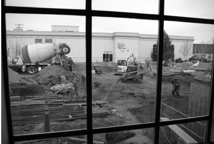
Looking north at the construction from the museum's administration offices.
