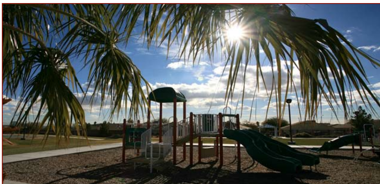
Petitti Park playground renovations.
