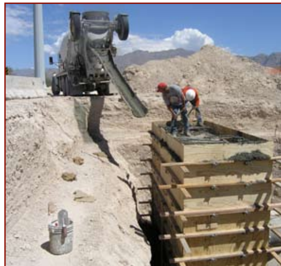
In-progress utility construction.
