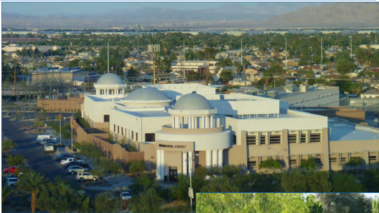
North Las Vegas Municipal Court and Justice Facility
