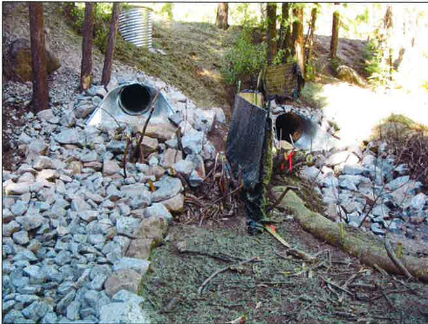
Rosewood Creek restored outfall
