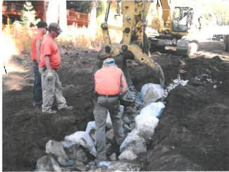
Building Channel during Phase 1 of the Rosewood Creek Area A SEZ Restoration
