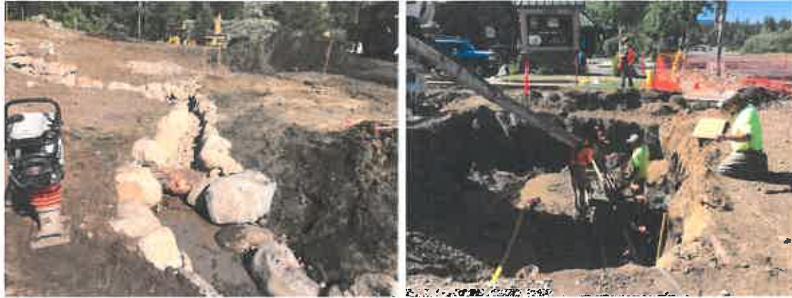
Construction on Burke Creek Crossing Project, September 2016
