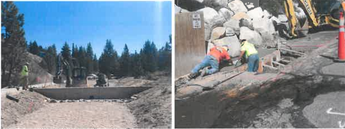
Construction on Cave Rock Erosion Control Project (Phase 1: left, Phase 2: right)
