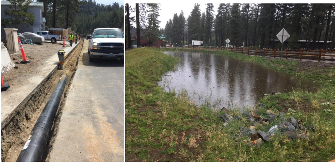
Zephyr Cove GID Water Quality Improvement Project: Left, installation of storm drain, Right, Newly constructed basin collecting runoff.
