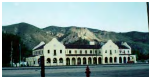
Caliente Branch (in southern part of building)
