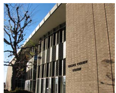
Washoe County Library
