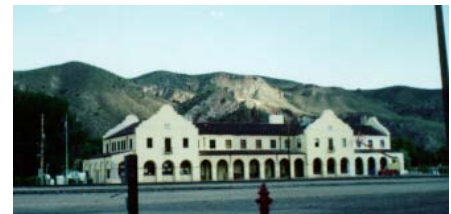
Caliente (part of old train depot)
