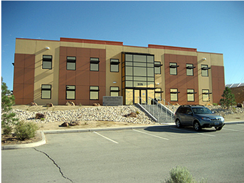
Photo 1. Nevada Bureau of Mines & Geology's new Great Basin Science Sample and Records Library on the campus of the Desert Research Institute.
