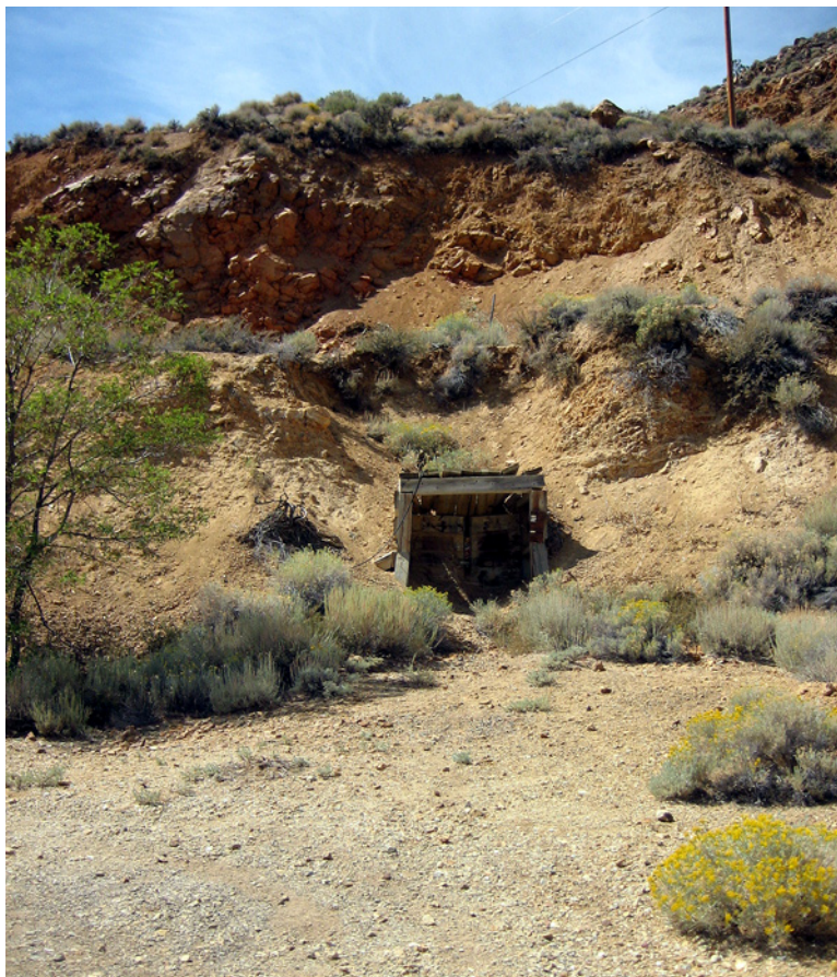
Photo 8. Closed mine adit at the Kendall Cut, Virginia City. “Stay Out and Stay Alive.”
