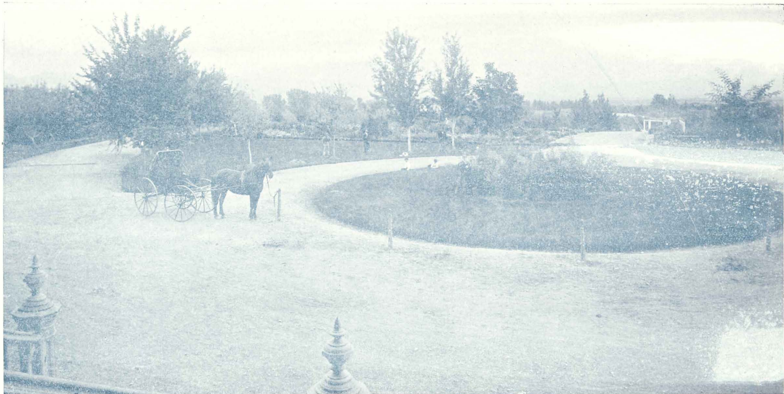
VIEW IN FRONT OF HOSPITAL.
