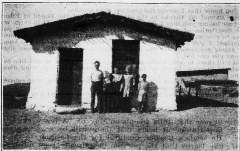
One type of rural school, built of mud and stone with willow roof.
