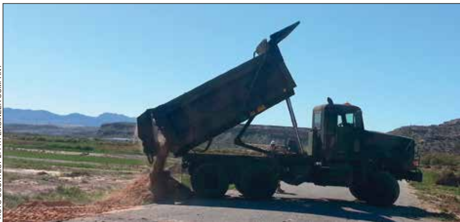
Sgt. Ryan Gillmore from the 777th Engineer Team directs a dump truck emptying a 20-ton load of dirt along a half-mile section of damaged levee and roadway washed out during flooding in southern Nevada. The engineers are assisting with the repairs at the Moapa Band of Paiutes reservation where the flooding damaged an earthen dam, levee and roads.
