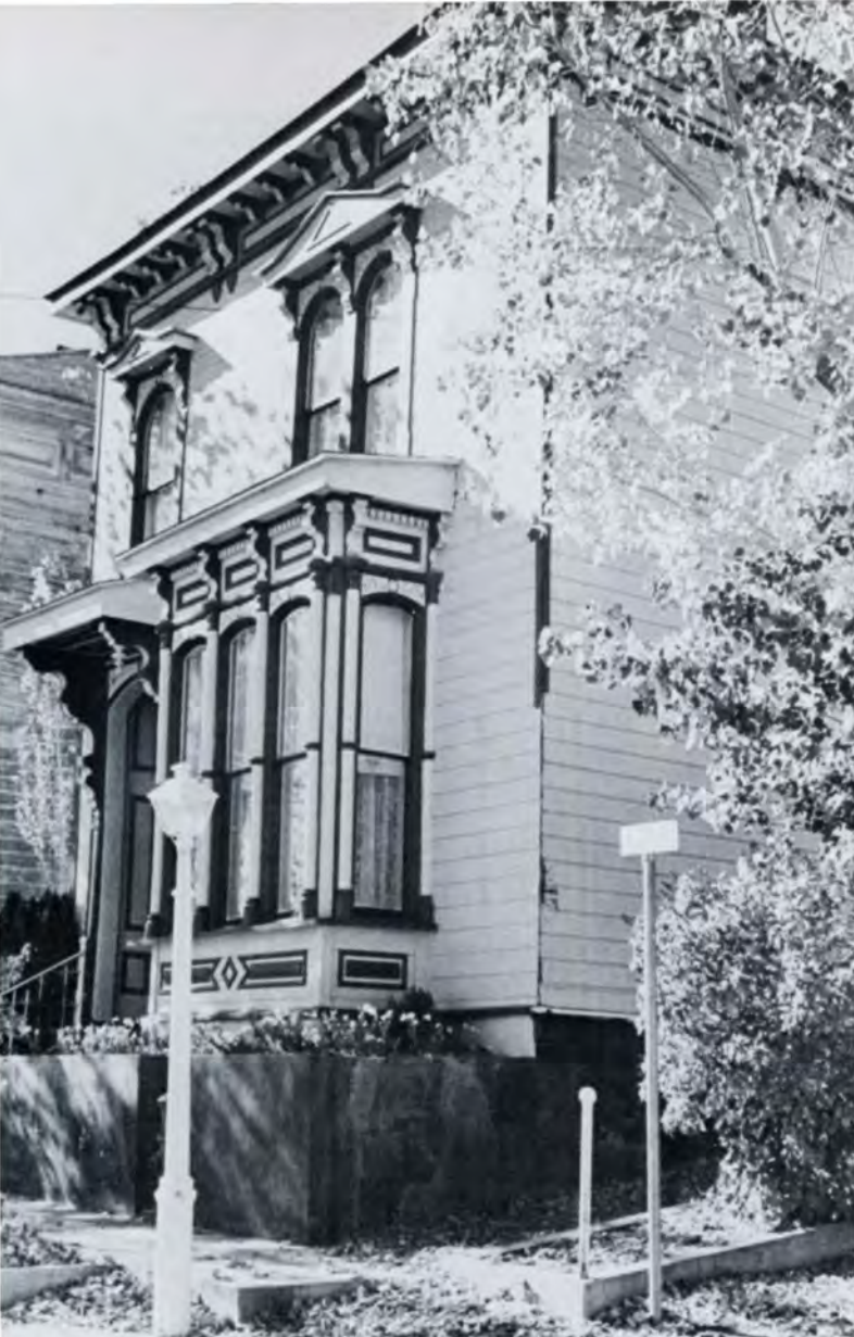
The Piper Home on A Street lay empty for many years until acquired and restored by Lucius Beebe, well known author of books on the early railroads and other Americana.
