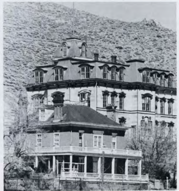
The Fourth Ward School forms a backdrop for the Chollar Mansion when viewed from the east. The school's cut-stone foundation is anchored to the solid granite of Sun Mountain by means of steel rods that tie its four stories to the foundation. Built in 1875 the school's last class was held in 1936. The Chollar Mansion on D Street is now closed to the public, but tours are still available into the Chollar Mine whose entrance is below and to the east of the mansion.
