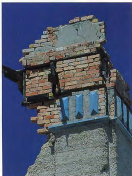
Brickwork teeters near the top of the John S. Cook Bank building.
