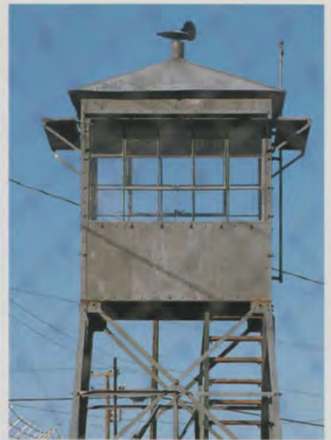
This Army Air Force observation tower now stands at the Tonopah museum.
