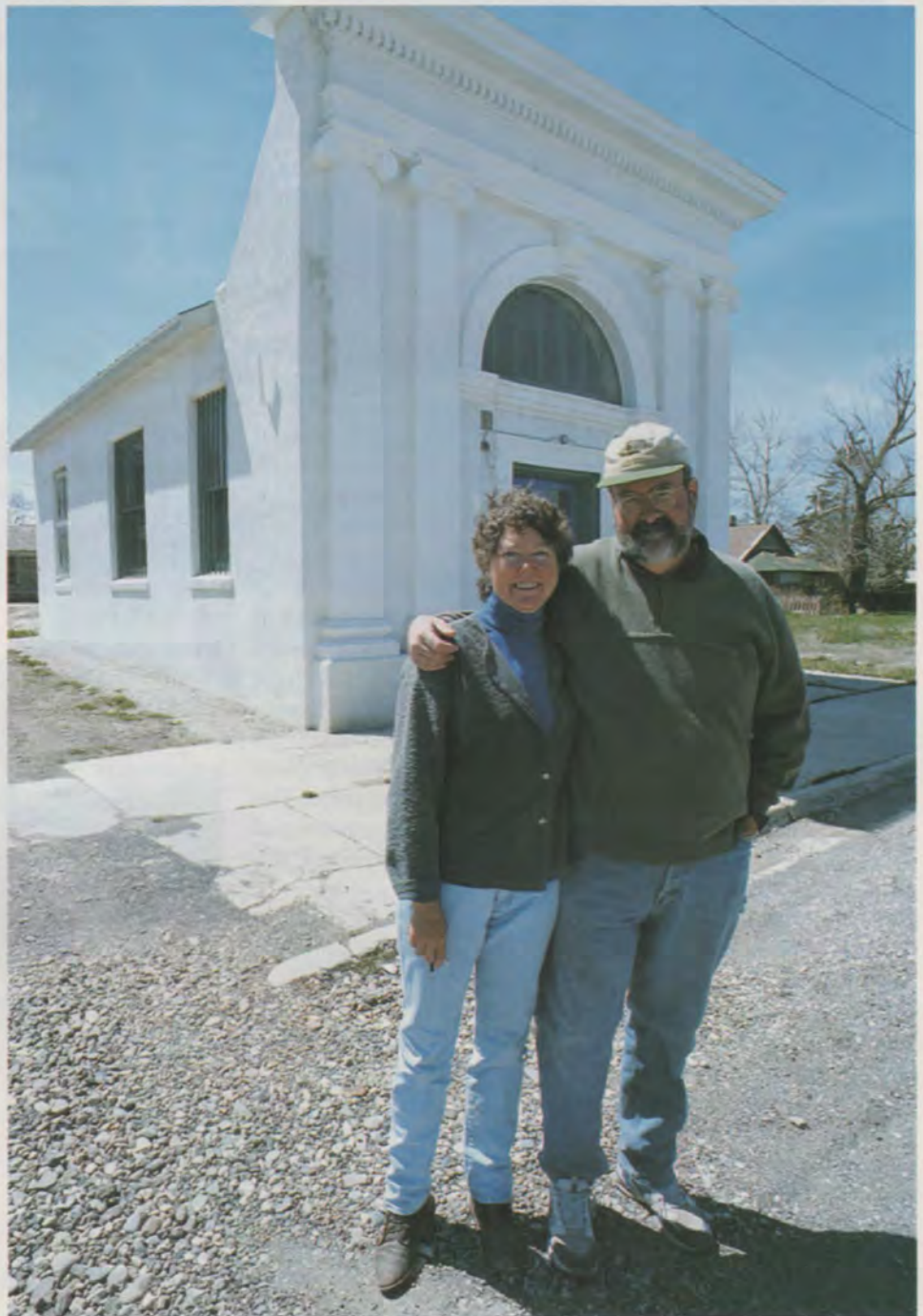
Jordan and Cannon stand in front of the historic Bank of Wells, which the couple bought and restored.
