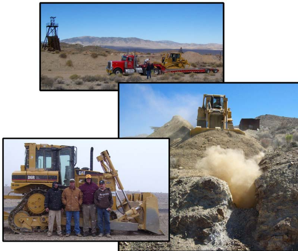
Figure 7. Southern Nevada backfill operations at Gold Point and Lida.
