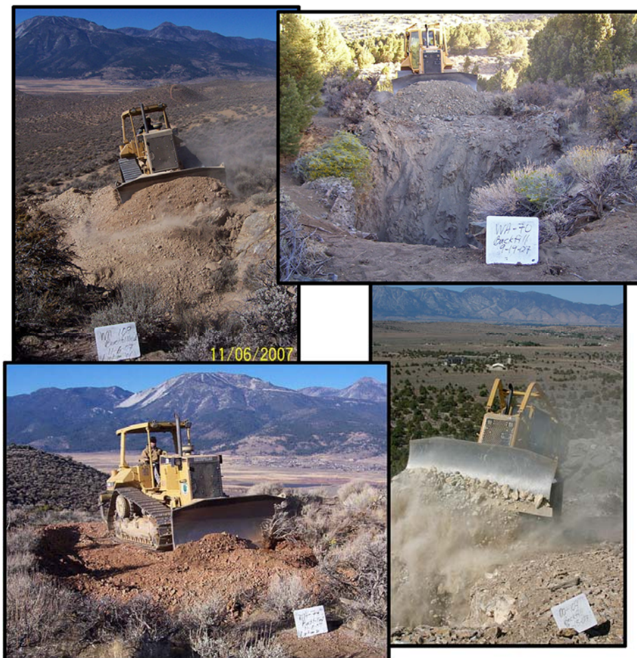
Figure 8. Backfill operations in Douglas and Washoe counties.
