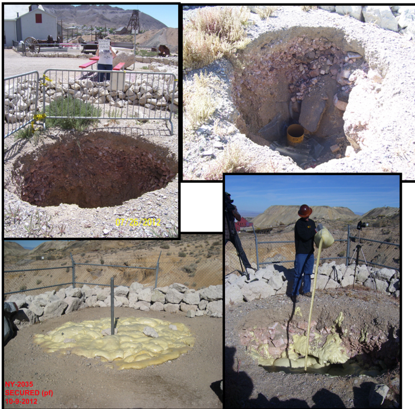
Figure 10. Polyurethane expansive foam (PUF) plug installed in the Mizpah air shaft at the Tonopah Historic Mining Park by Environmental Protection Services.
