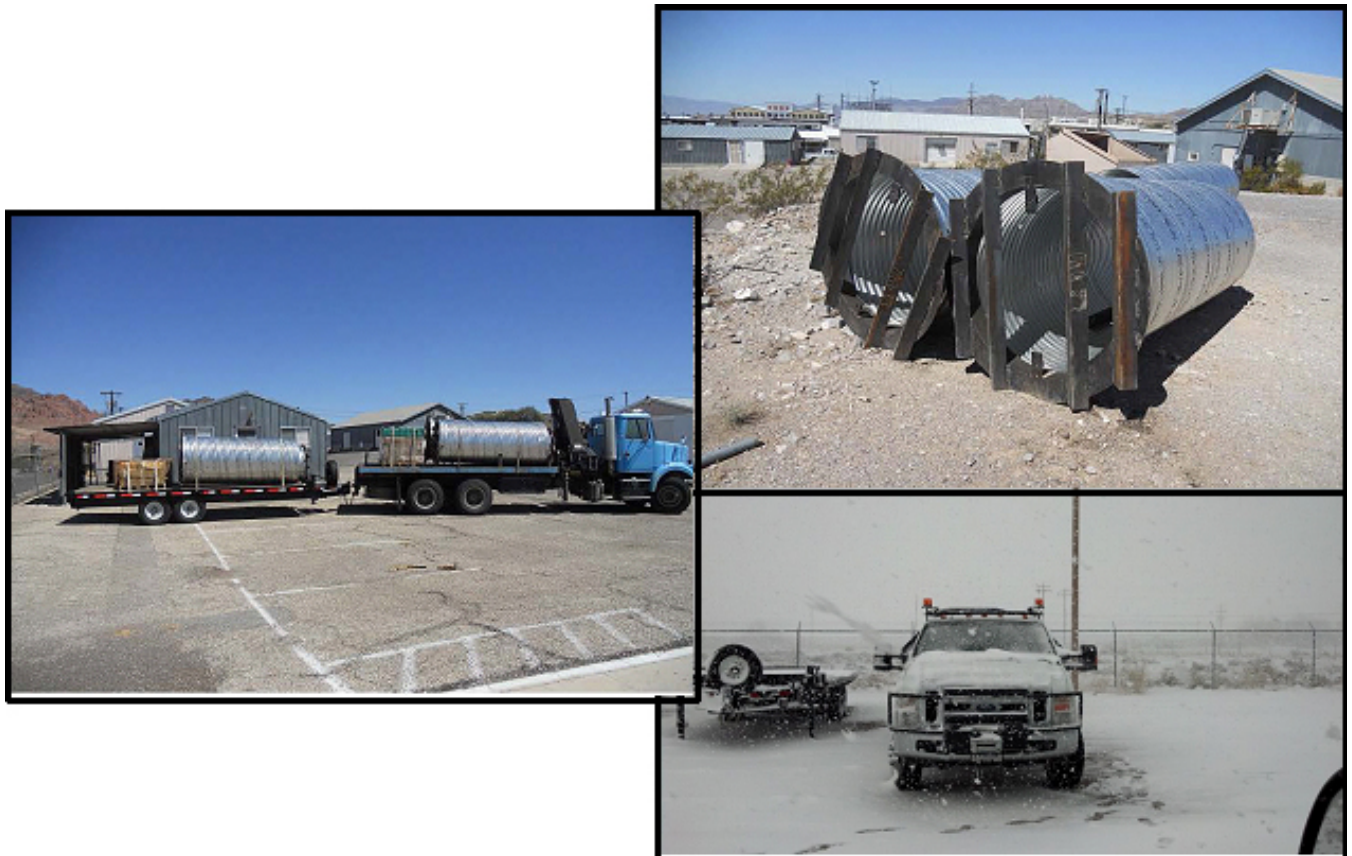
Figure 7. Bureau of Reclamation (BOR) preparation and mine closure work in Clark and White Pine Counties. Clockwise from left: Truck loaded with PUF and prepped culvert gates; culvert gates ready to install; winter storm in White Pine County.
