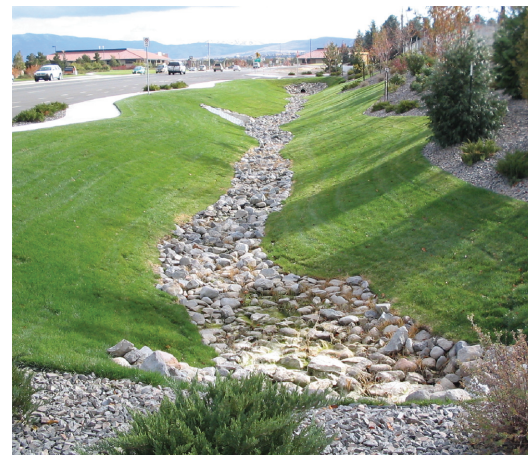
A vegetated swale is an example of a storm water structural control feature.
