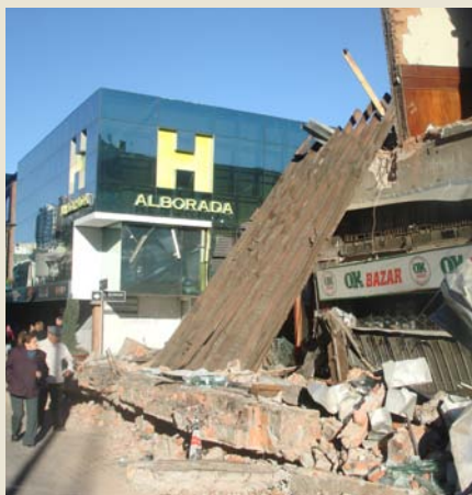
Engineering faculty member Gokhan Pekcan took this picture of damage from the magnitude 8.8 Feb. 27 earthquake in Concepcion, Chile’s second largest city. It shows differences in damage between old construction methods and construction that follows new national building code standards.
