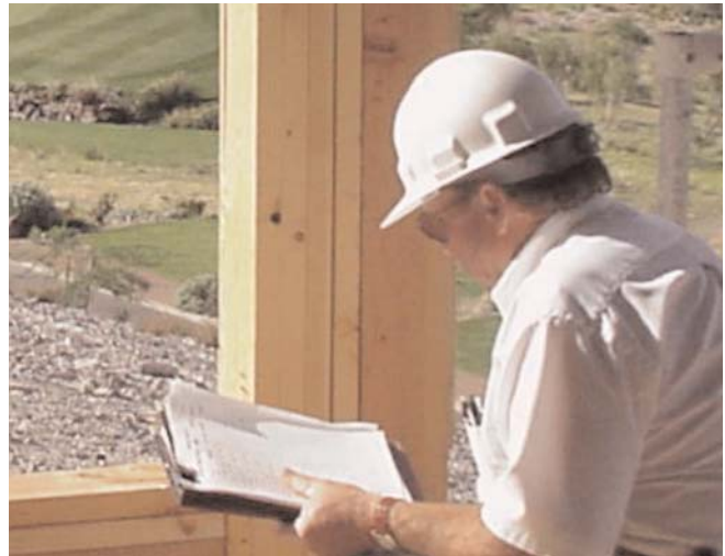
New Construction Inspection
