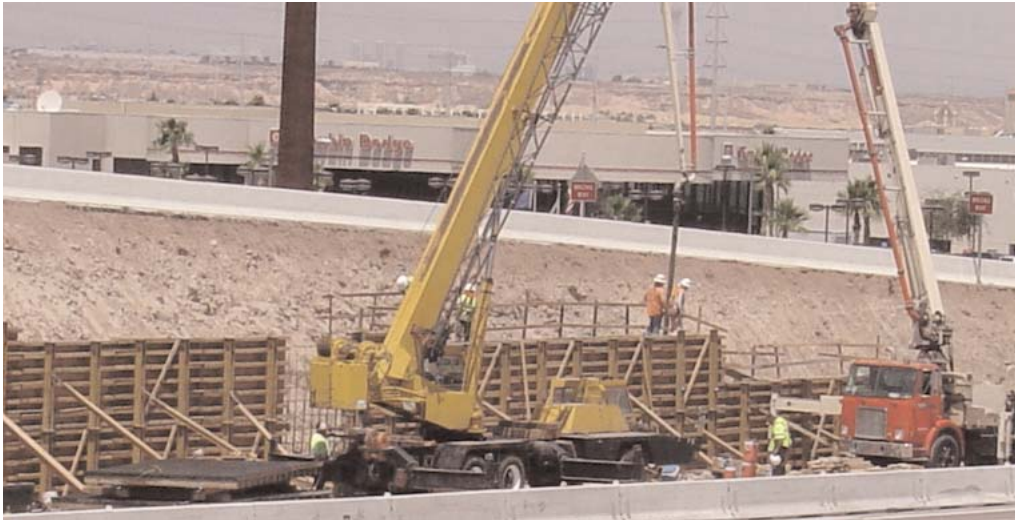
Autoshow Rd/I515 Interchange Construction
