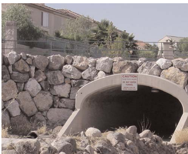
Seven Hills Flood Control
