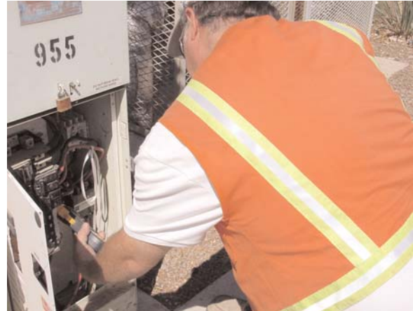
Streetlight Control Panel Repair
