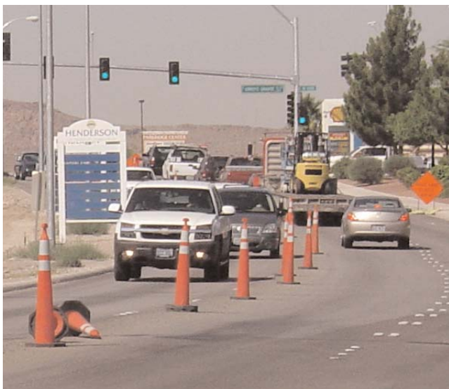
Horizon Ridge Parkway Construction
