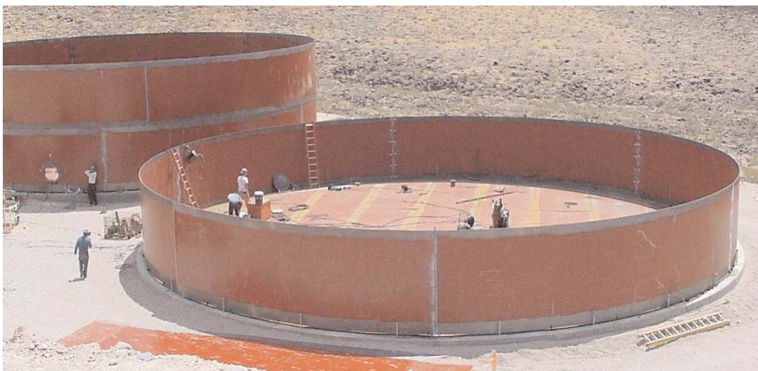
New Reservoir Construction
