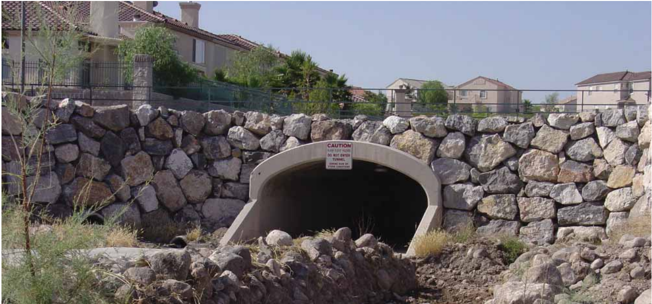
Seven Hills Flood Control
