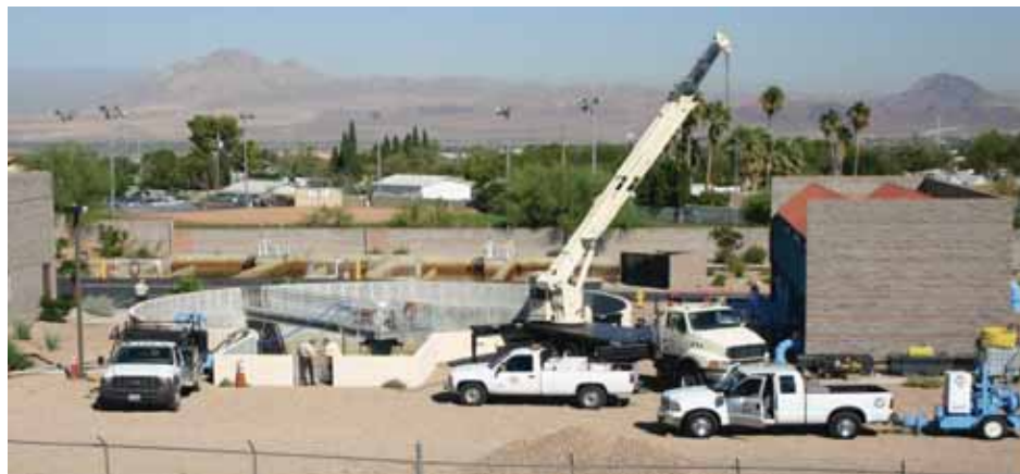
Backflow Recover Basin Maintenance
