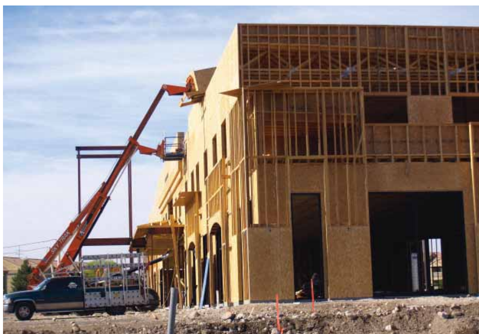
Commercial Building Site
