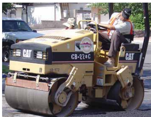
Street Patch Repair
