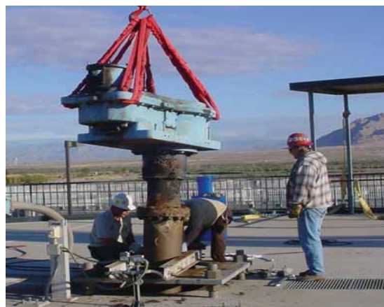
Gearbox Replacement at WRF Aerator
