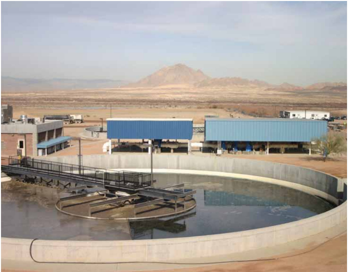
Water Reclamation Facility Expansion
