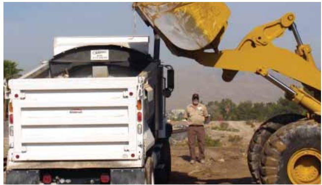
Public Works Crew at Project Site
