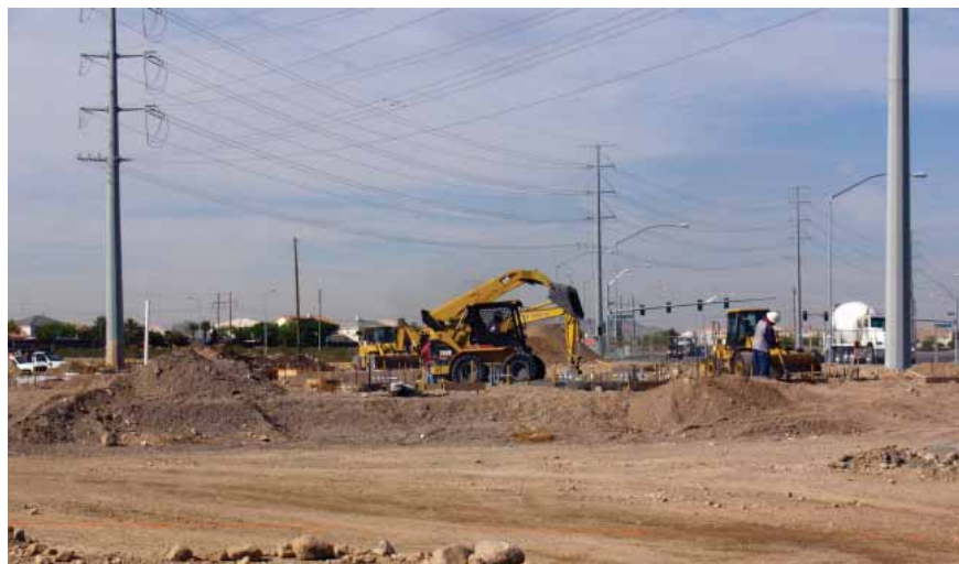
New Construction Project
