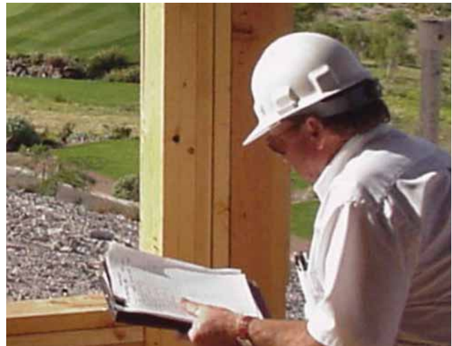
New Construction Inspection
