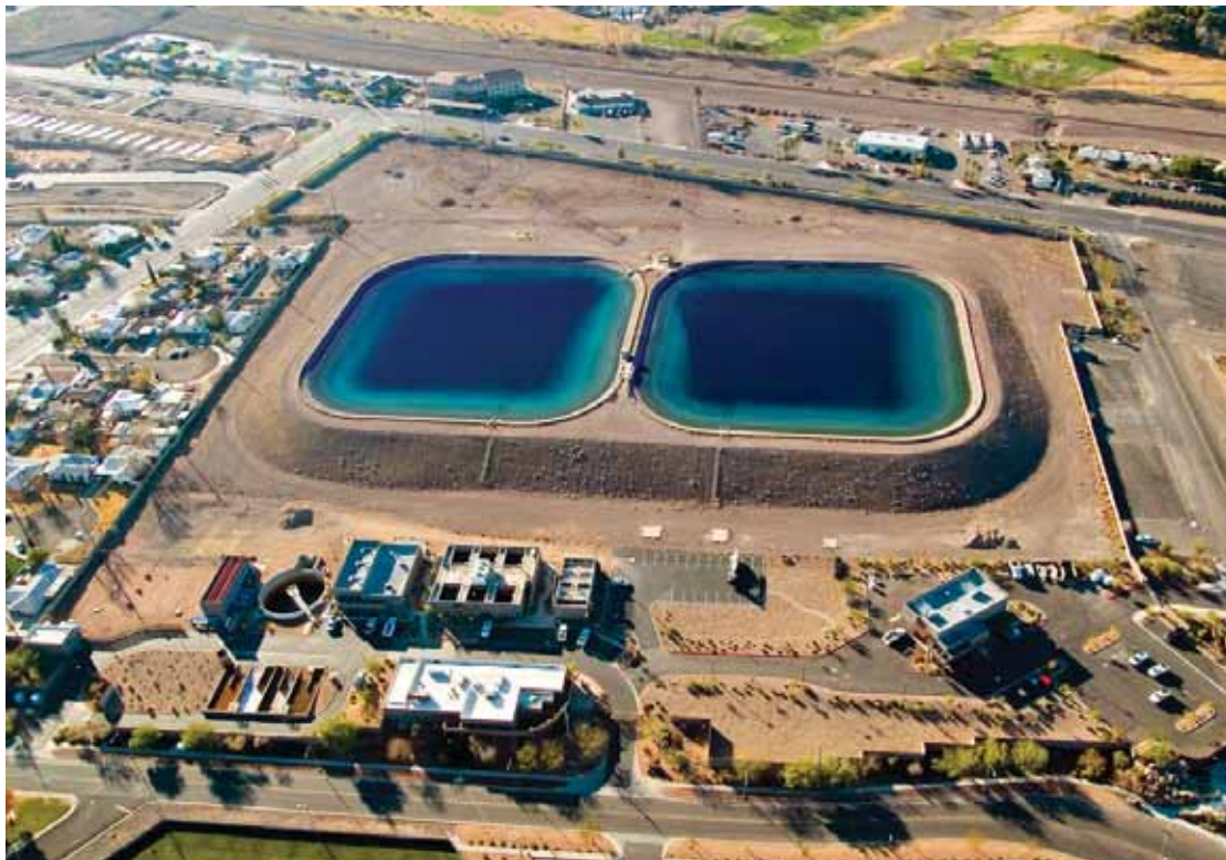
Water Treatment Plant Facility
