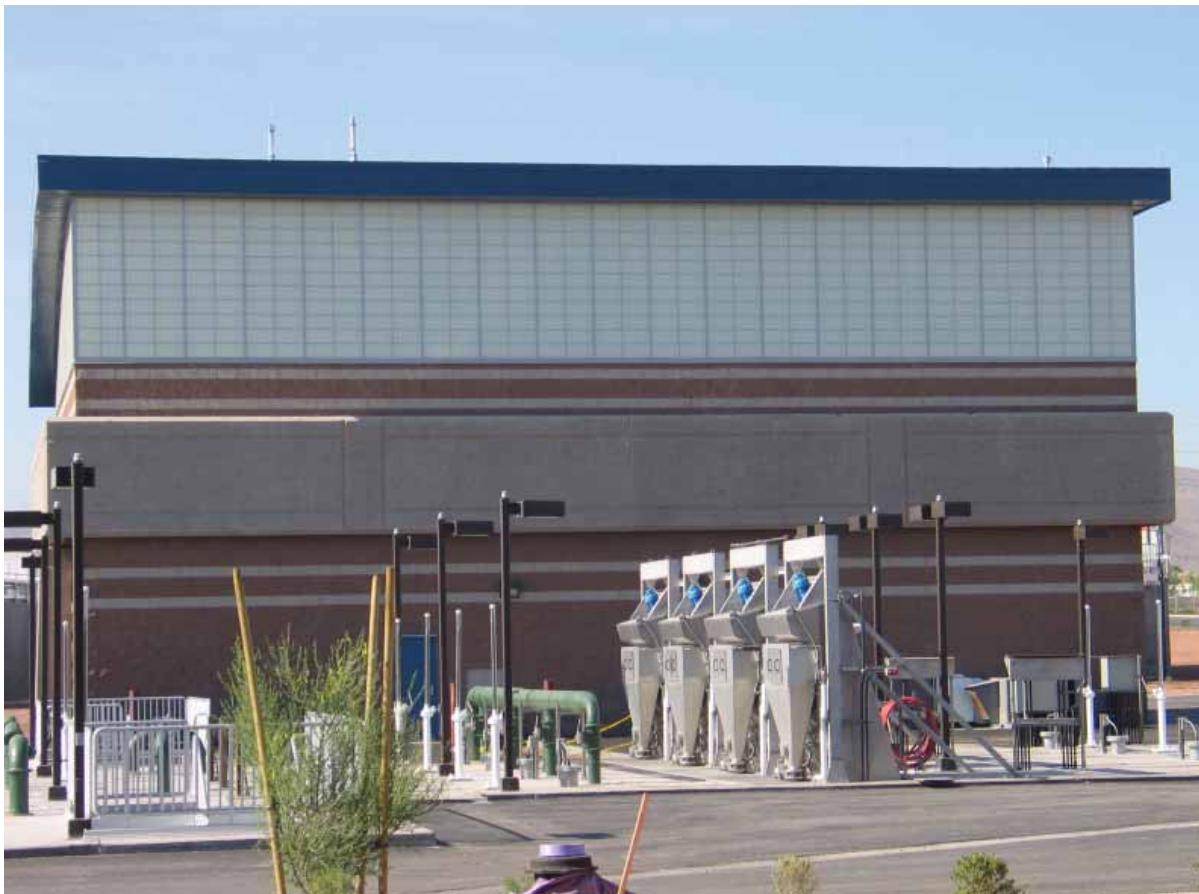
Water Reclamation Facility
