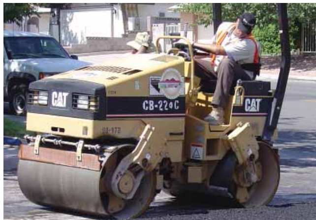
Street Patch Repair
