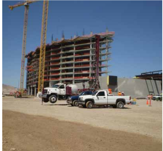
M Resort Under Construction
