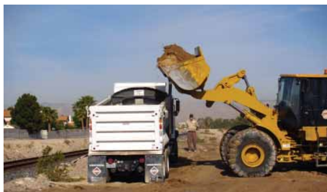
Public Works Crew at Project Site
