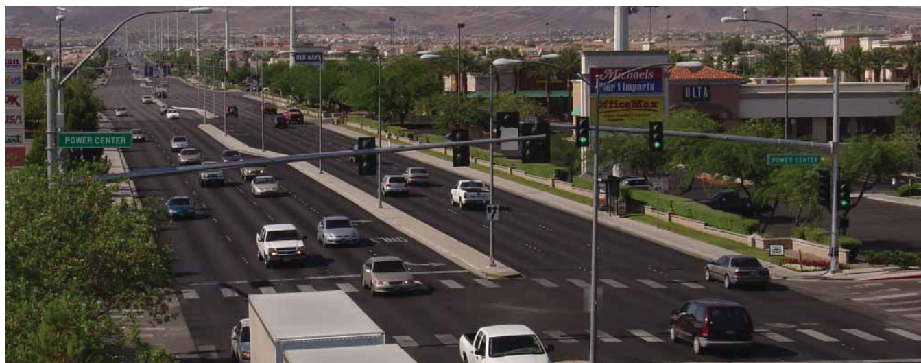
Stephanie Street Rehabilitation
