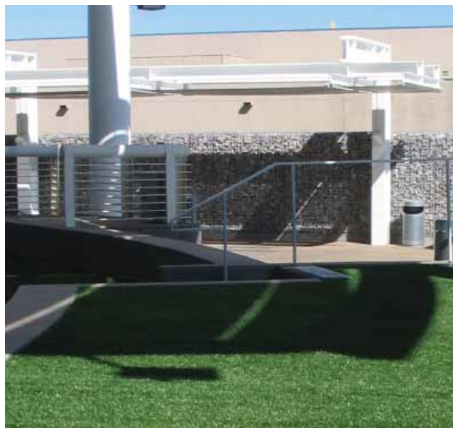
Artificial Turf Utilized at the Events Center Amphitheatre for Water Conservation
