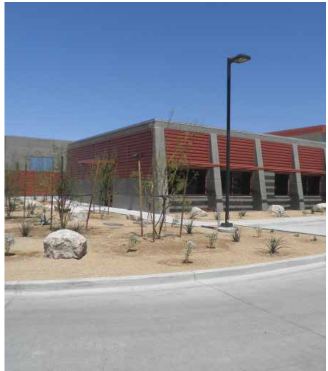
The Southwest Water Reclamation Facility began operating in December, 2011 and adds approximately 8 million gallons per day capacity to existing treatment.
