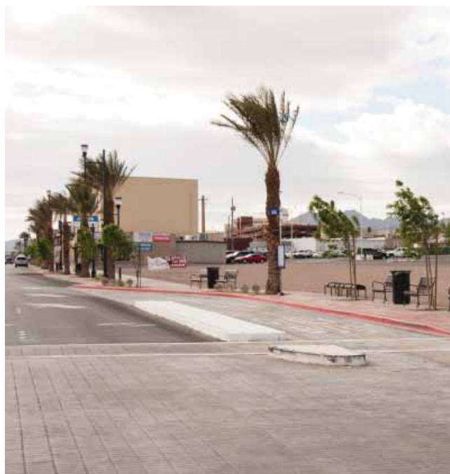
Water Street Improvements
