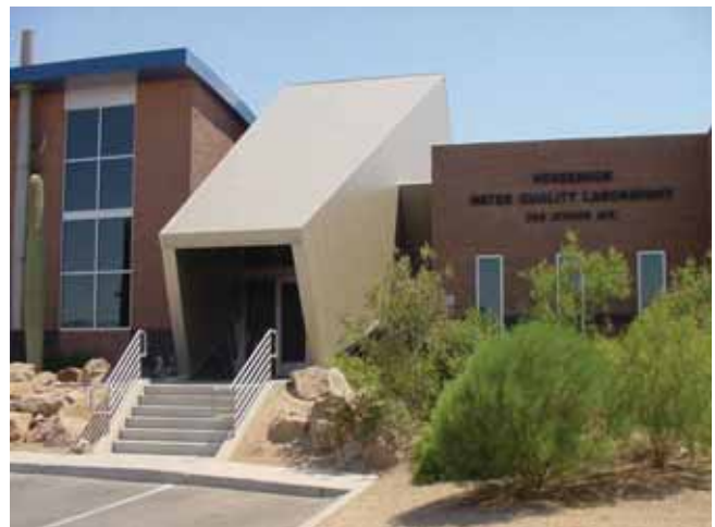
Laboratory Facility on Water Reclamation Facility Campus
