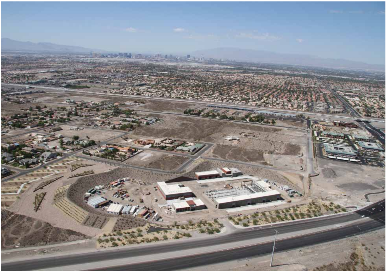
Southwest Water Reclamation Facility
