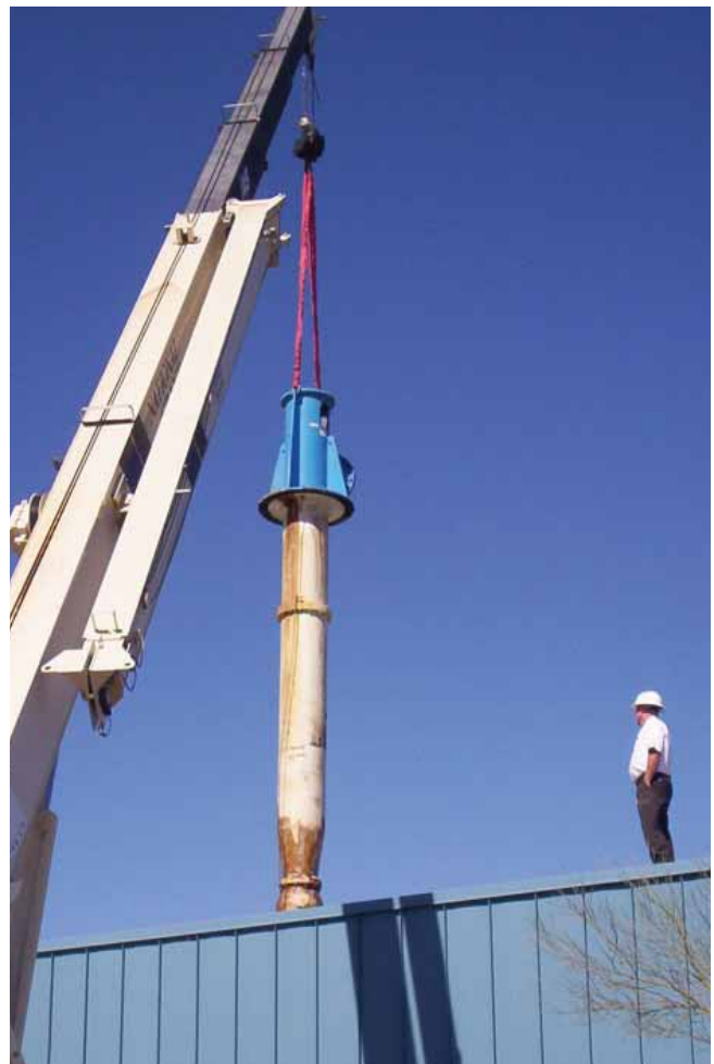
Reclaimed Water Pump Removal
