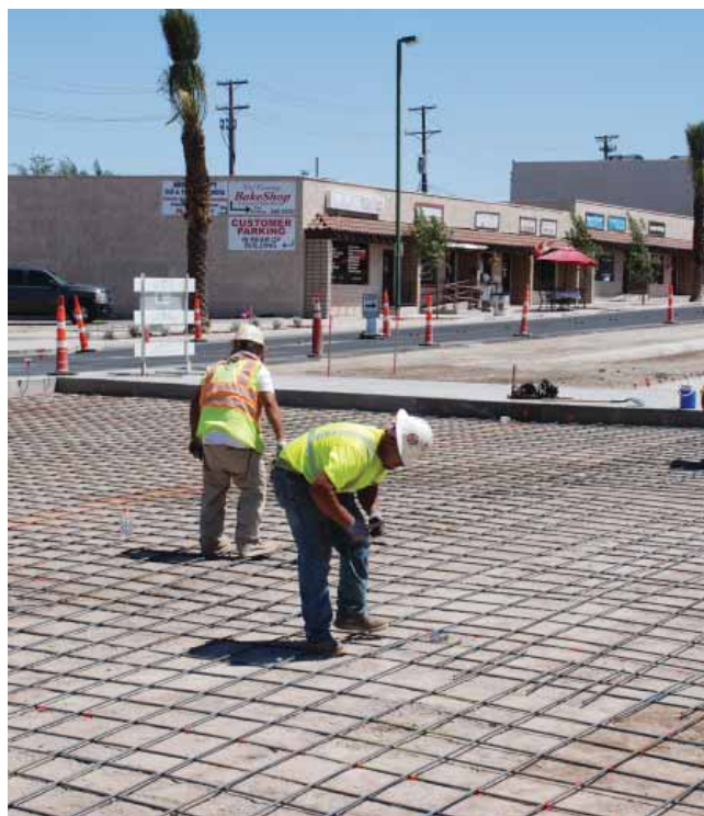
Water Street Improvements
