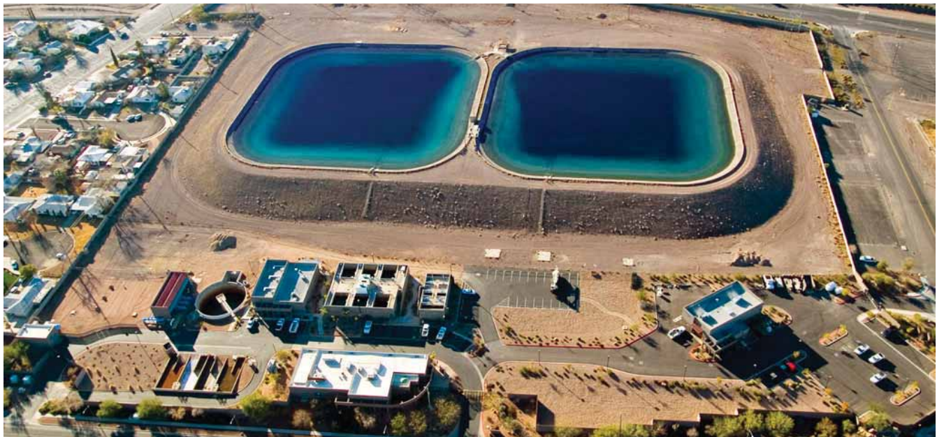
Water Treatment Plant Facility
