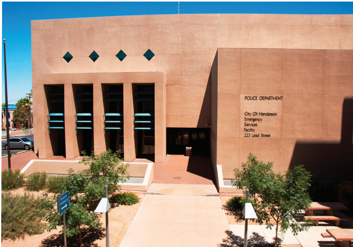
Emergency Services Building
