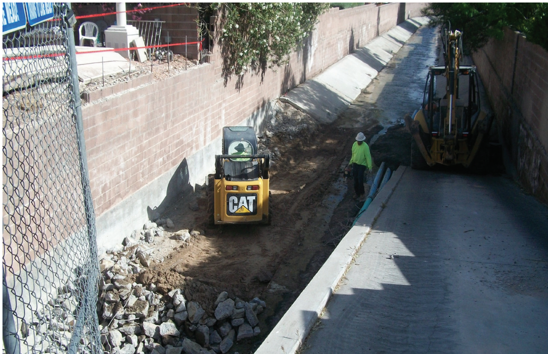
Whitney Ranch flood control channel repairs
