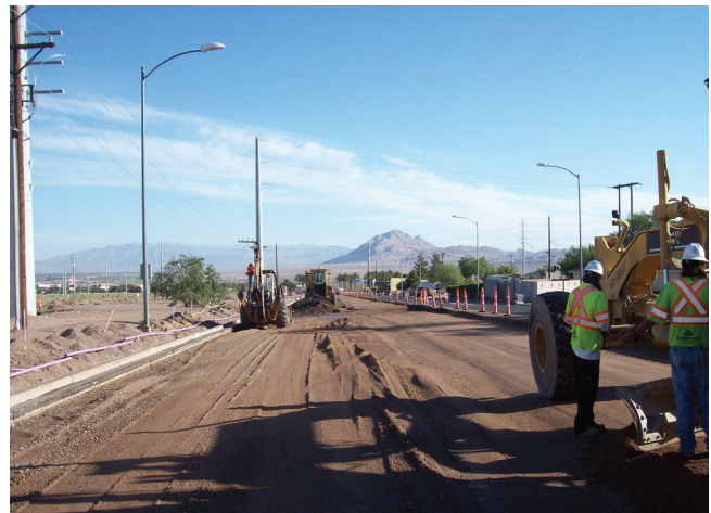
Water Street replacement Lake Mead to Boulder Highway
