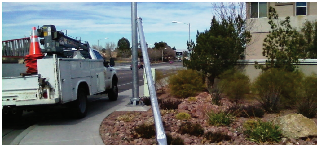
Street Pole Replacement
