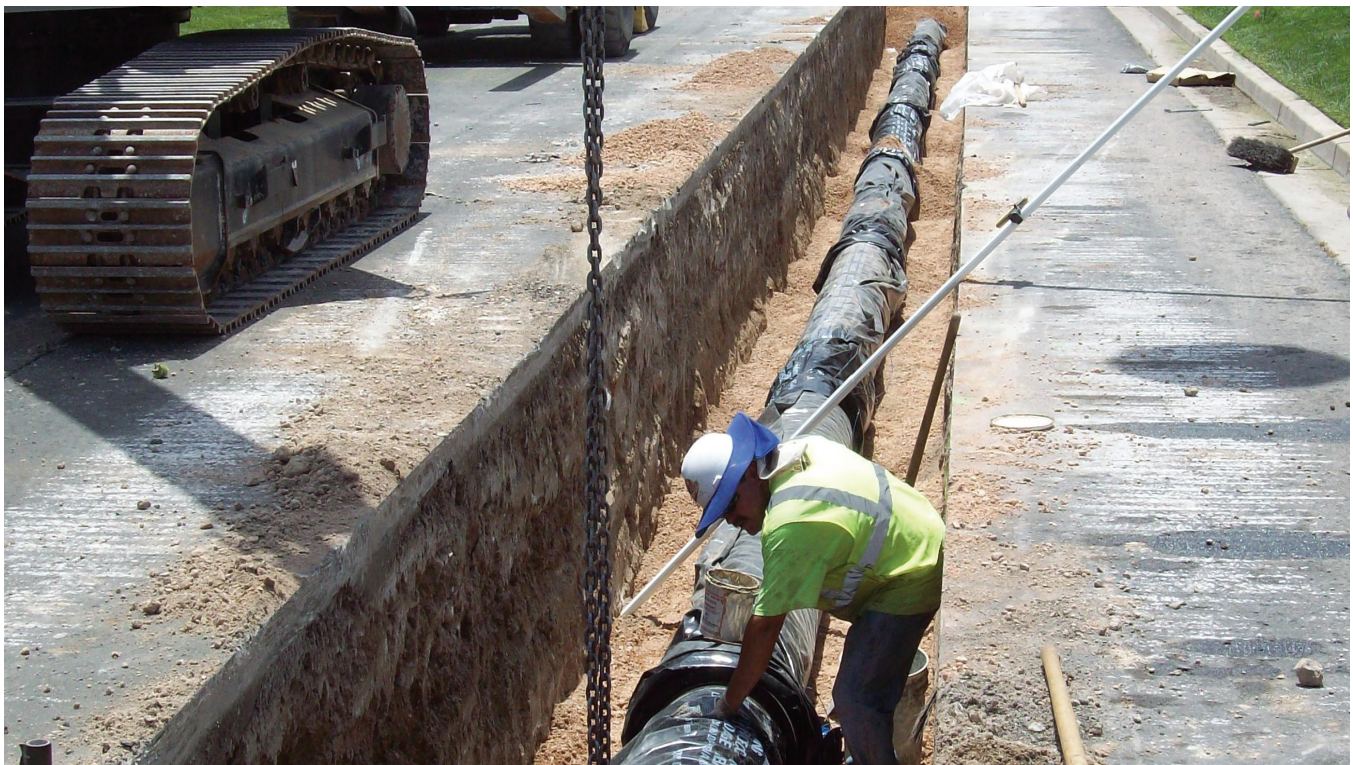
Installing 16 inch water lines
