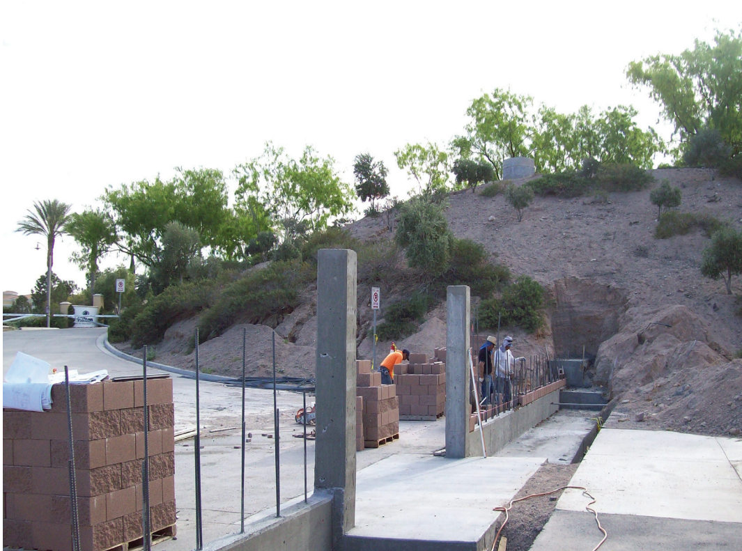
Block wall construction
