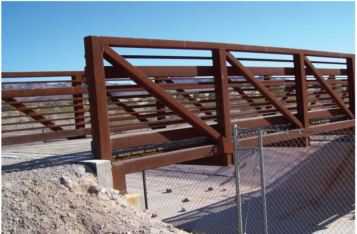
Equestrian Detention Basin
