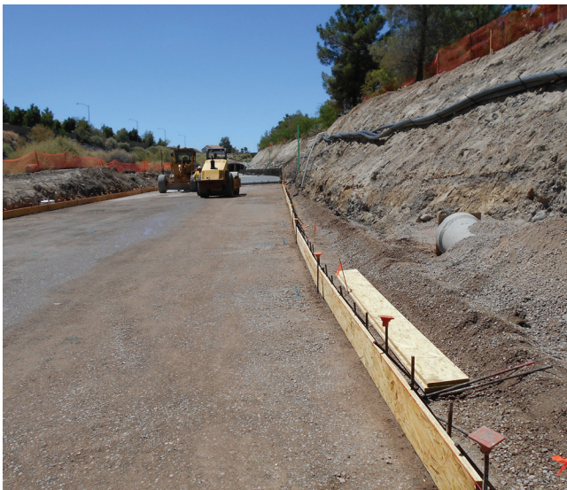
Work on Pittman Wash
