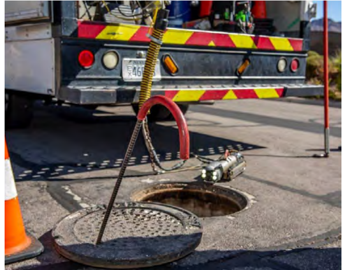
Field Operations assessing a sewer line
