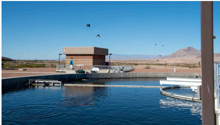
Water Reclamation Facility
