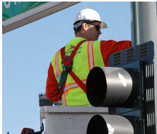
Street light repair
