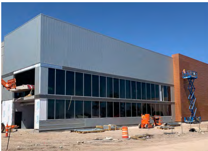
Construction on the new Golden Knights' Lifeguard Arena practice facility and community ice rink
