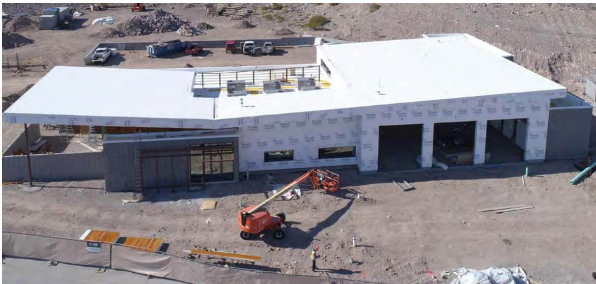
Aerial view during the construction of Hidden Falls Fire Station
