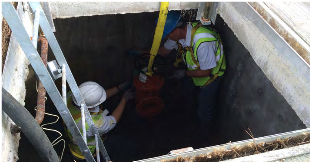
Utility staff working on a large meter
