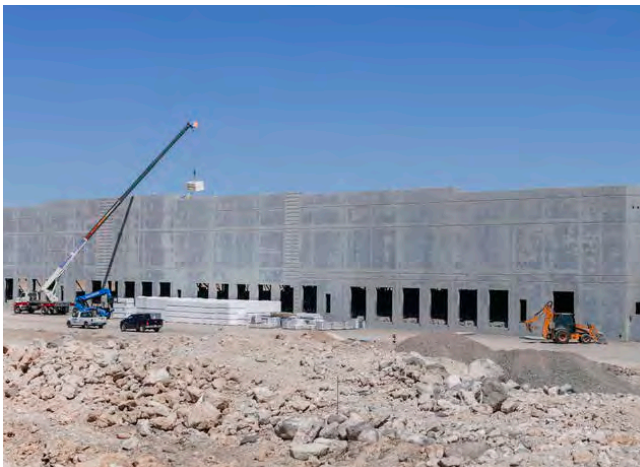
Construction on Amazon Distribution Center
