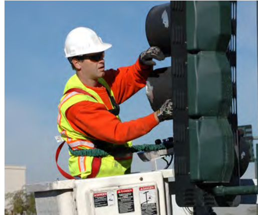
Traffic light repair
