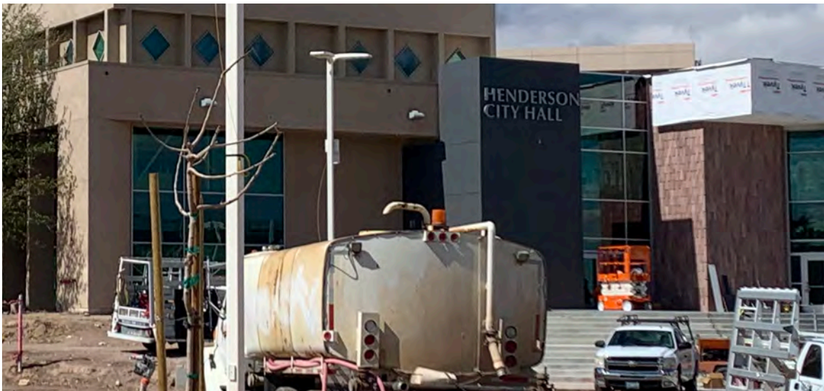
Construction of the Events Plaza and City Hall entryway
