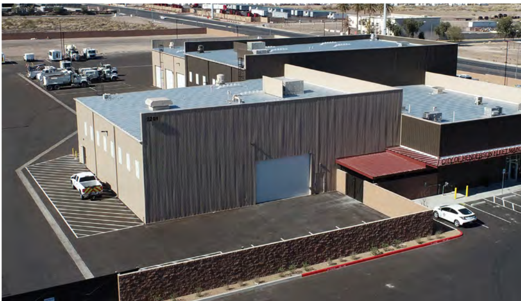
City of Henderson fleet maintenance building
