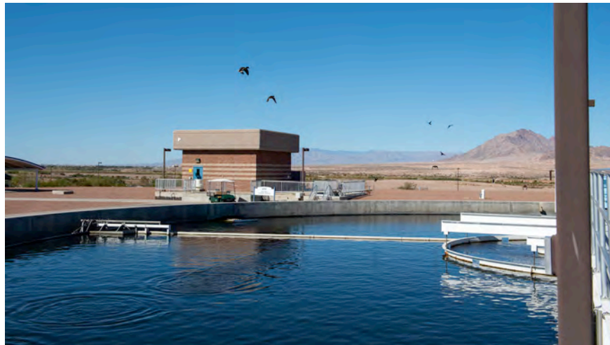
Water Reclamation Facility
