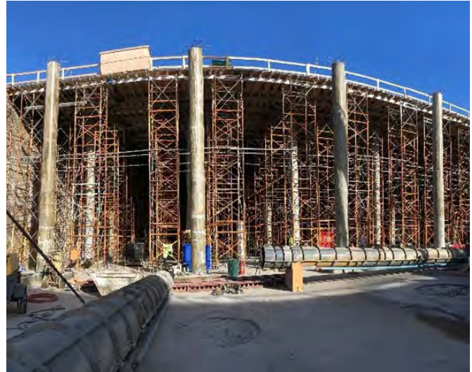
Construction of R-8 Reservoir
