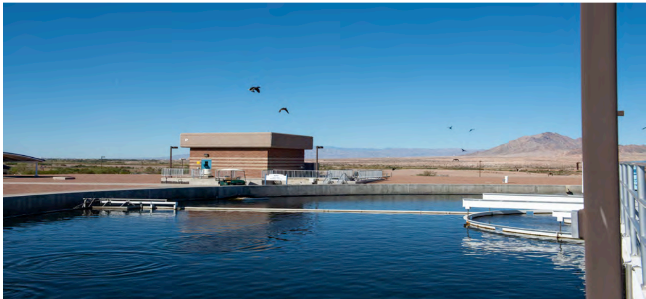
Kurt Segler Water Reclamation Facility
