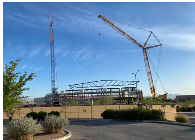
Dollar Loan Center construction
