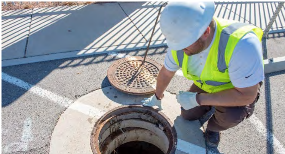
Pretreatment Inspector checking a manhole for gases
