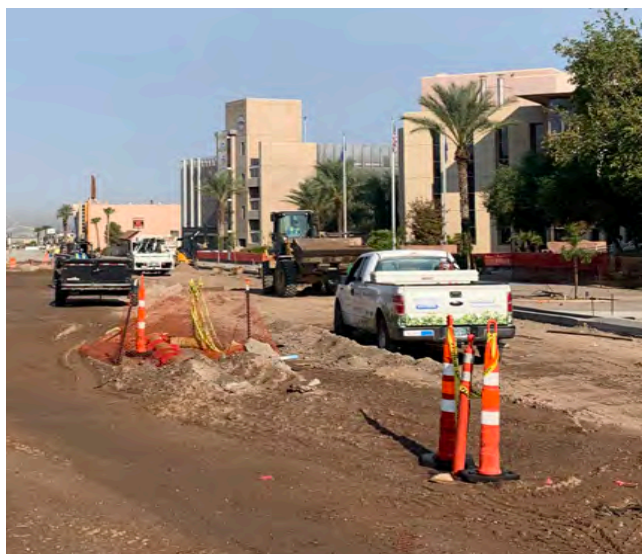
Road construction in the Historic Water Street District
