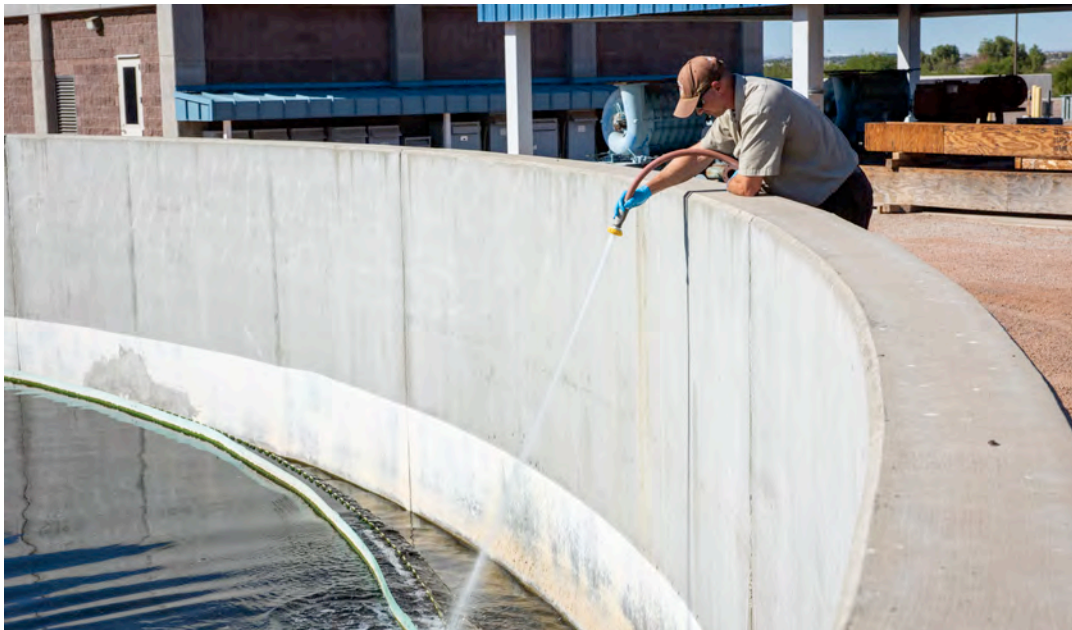
Wastewater Facilities Operator working at the Wastewater Recovery Facility
