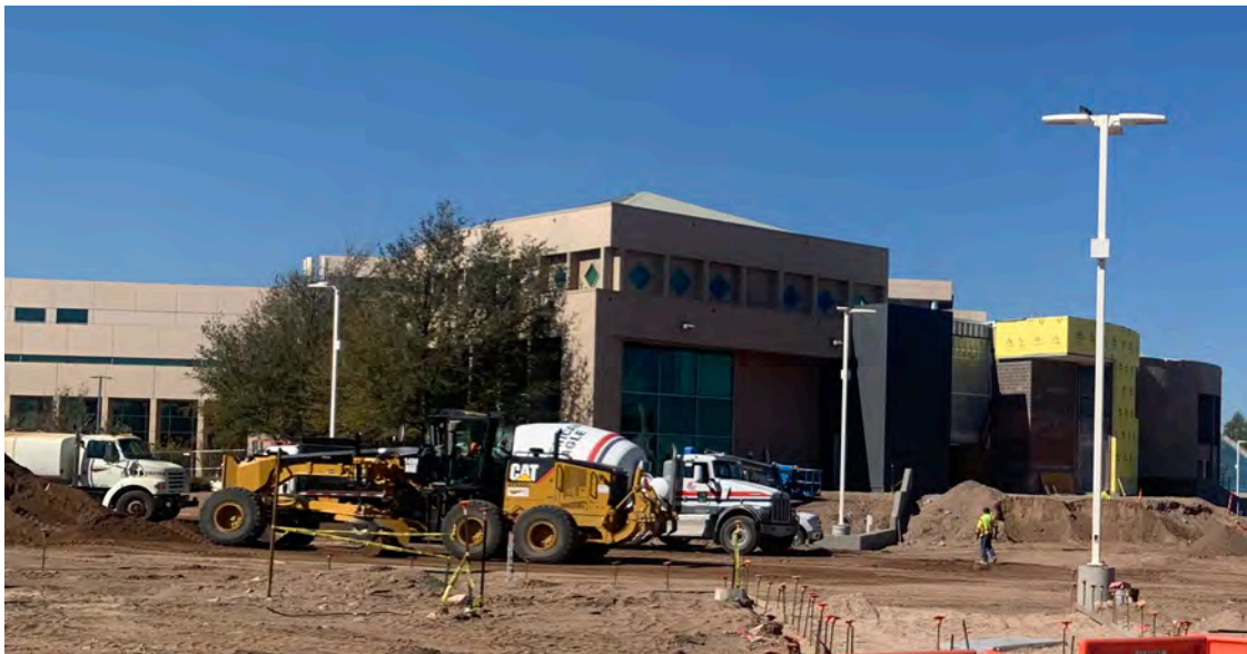
Building improvements to east City Hall entrance
