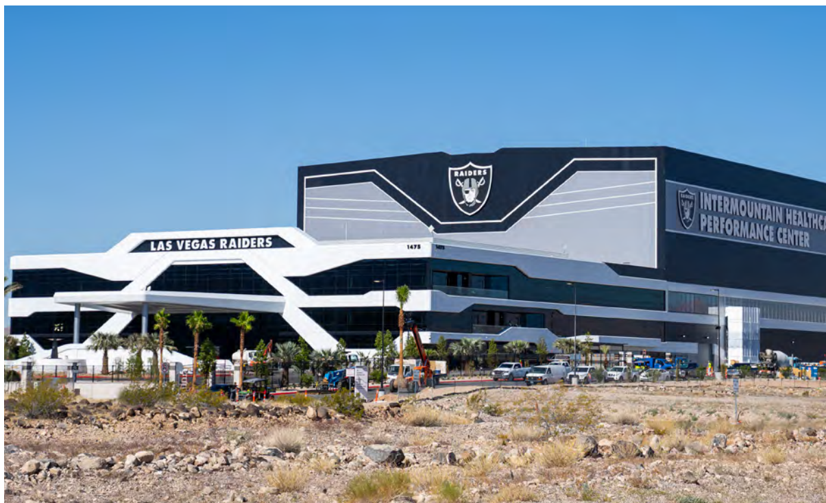
Las Vegas Raiders corporate headquarters and practice facility in West Henderson
