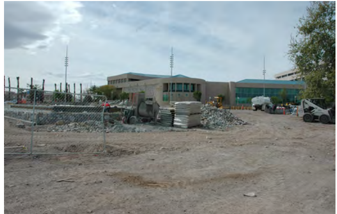
Construction of Water Street/Events Plaza improvements
