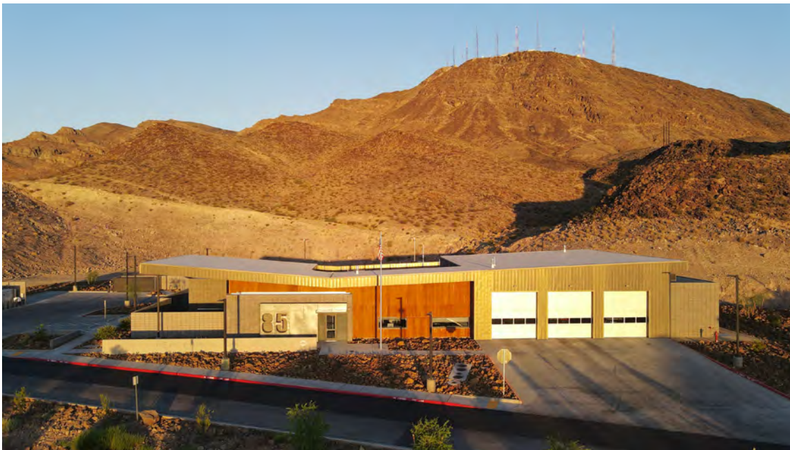
Fire Station 85, the City's 11th fire station was completed in Fiscal Year 2021
