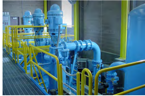
Water Reclamation Facility
