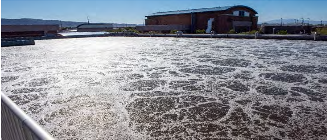
Water Reclamation Facility (WRF) Pond
