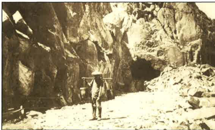
Heading (top cut) of East Portal, Tunnel No. 8
