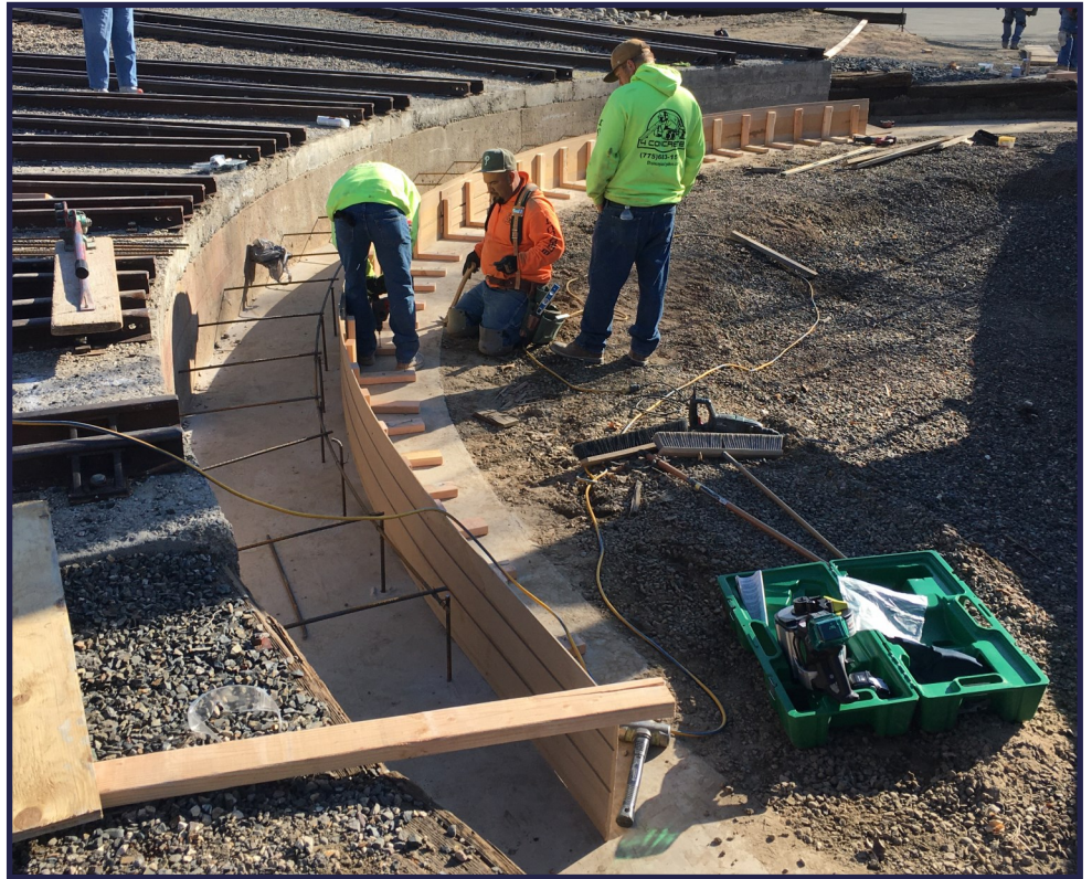
(Above) Workers from 4Concrete build the forms for the landing pad on the north side of the turntable nearest the Annex.
