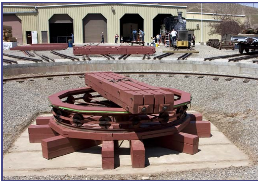
The pivot during the 2010 rebuild of the NSRM turntable. (NSRM photo)
