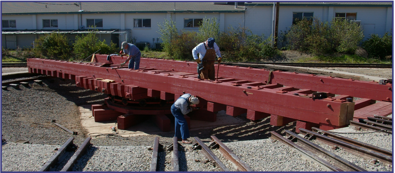
NSRM volunteers set to work installing the rebuilt turntable in 2010. (NSRM photo)
