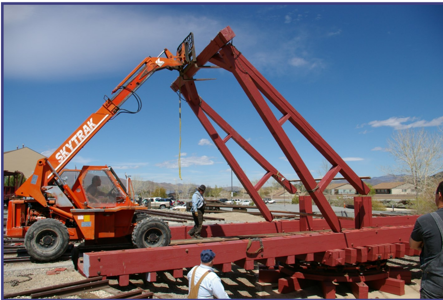
Hoisting the A-frame for the turntable in 2010. The original A-frame was reused and not rebuilt. (NSRM photo)
