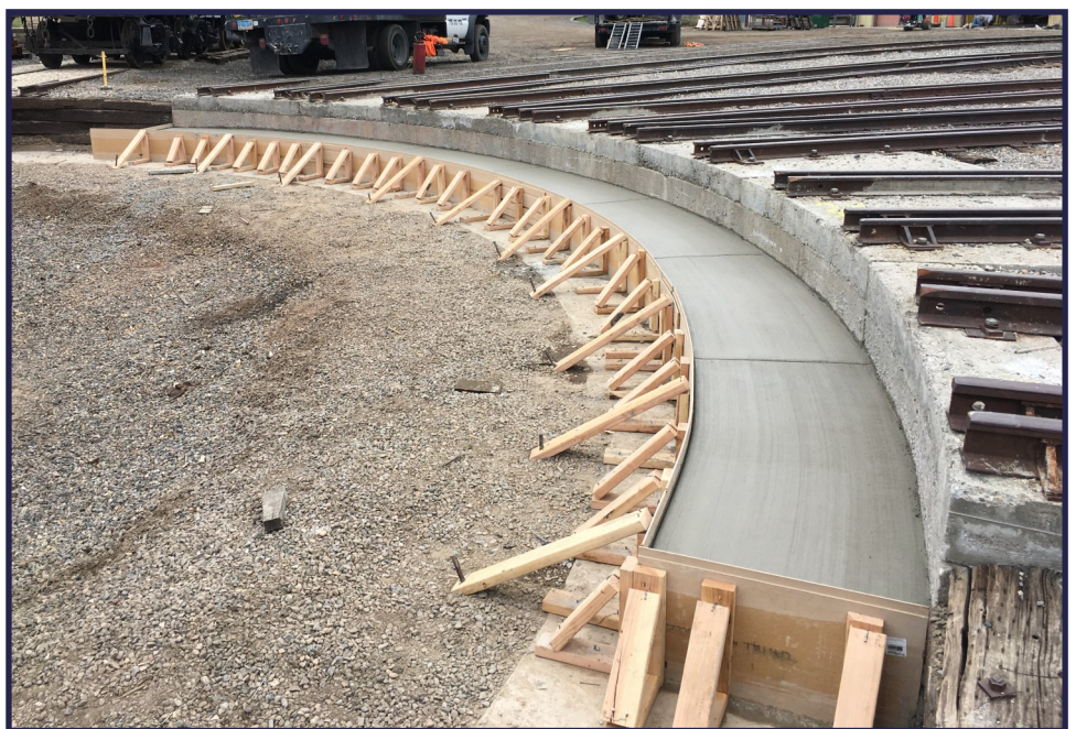
(Below) Later in the day, workers poured and formed the concrete into a landing pad. (NSRM photos)
