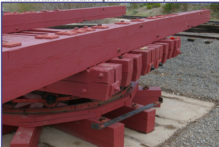
The side sills are added to the turntable during the 2010 rebuild. (NSRM photo)
