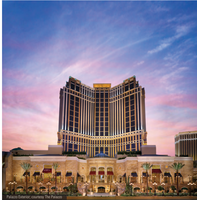
Palazzo Exterior, courtesy The Palazzo
