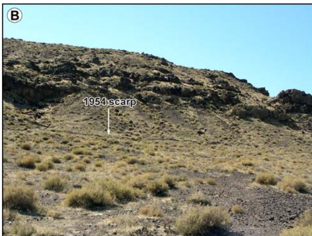
Figure 12. Surface ruptures produced by the 1954 Rainbow Mountain-Stillwater earthquakes. 12A. Small (30 cm) vertical 1954 scarp; photograph was taken by Karl Steinbrugge in late (?) 1954 near the Rainbow Canyon trench location of Caskey et al. (2004). 12B. Trace of ½-m-high 1954 scarp which is highlighted by shadow and lies along the trace of the east-dipping range-front fault bounding the east margin of Rainbow Mountain.
