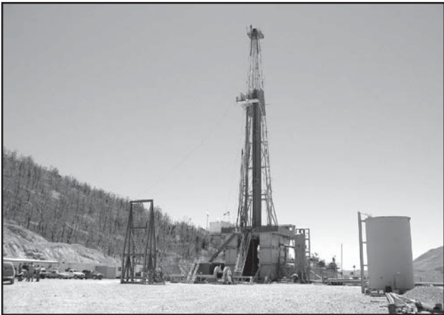
Drilling rig in the Piñon Range (Jon Price photo).
