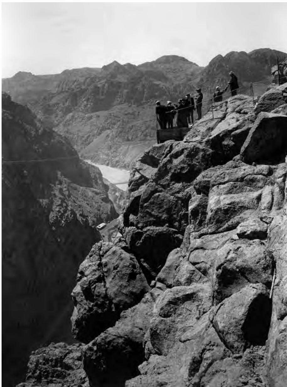
Figure 2. Visitors to the Boulder Dam construction site view Black Canyon from Lookout Point in April 1932. Photographer unknown. ( Special Collections, University Libraries, University of Nevada, Las Vegas )
