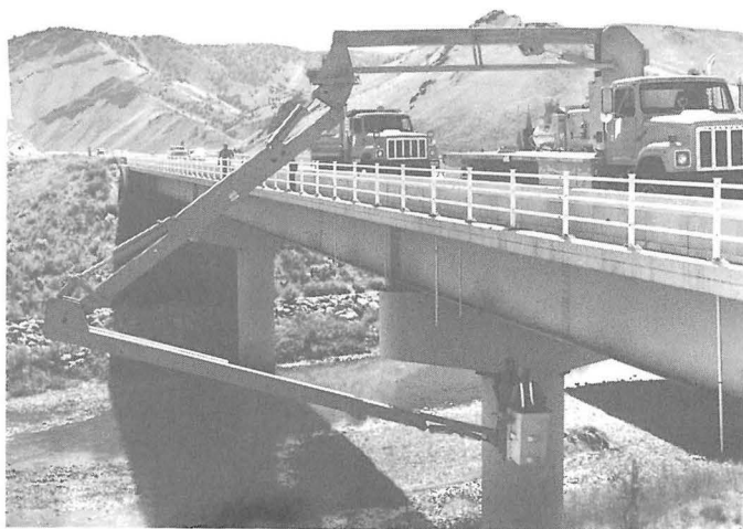
Inspecting a bridge over the Humboldt River
