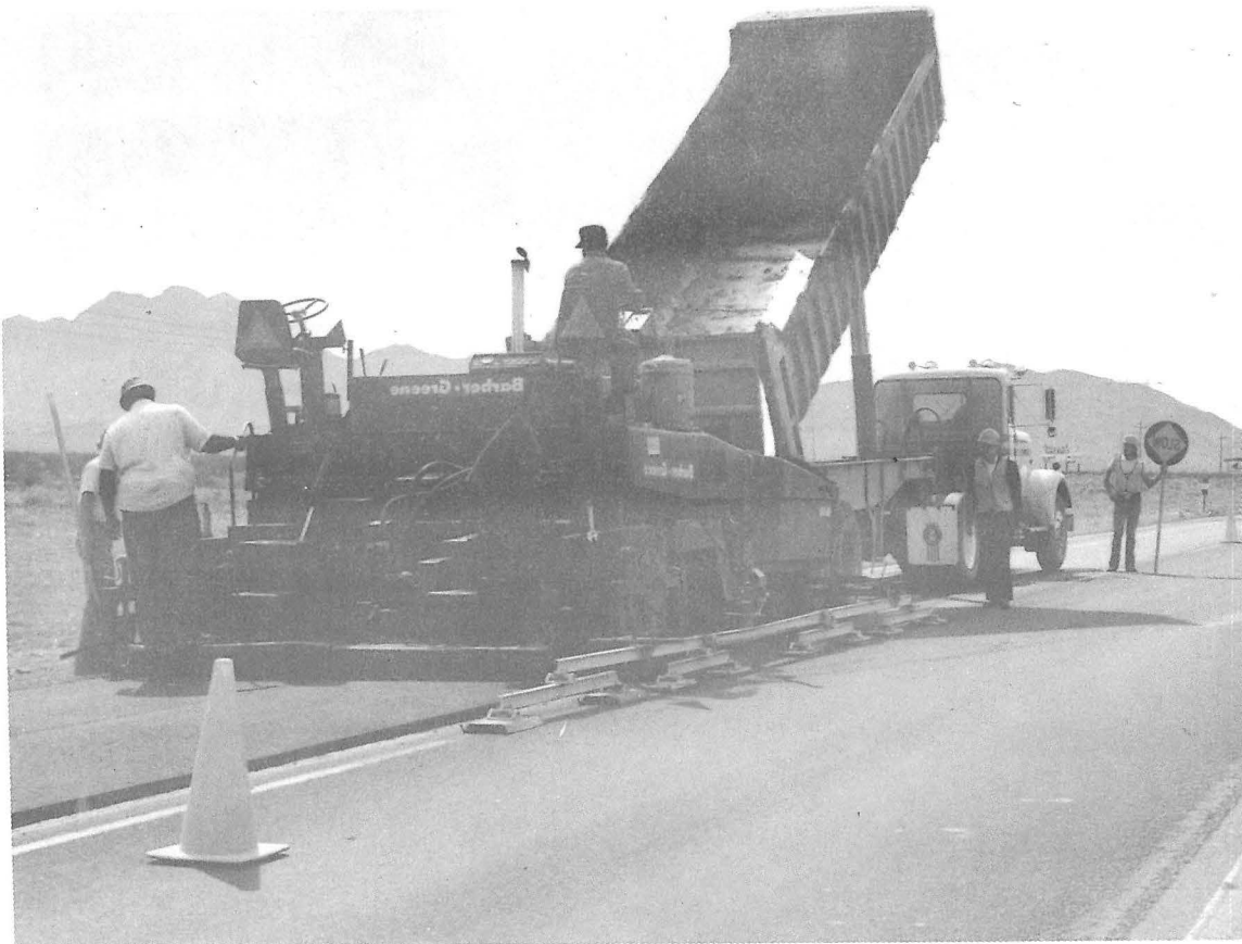
Placing a 2-inch minimum pavement overlay
