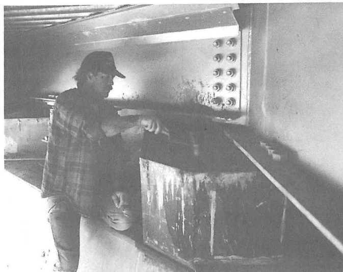
Seismic retrofitting on a bridge in Verdi
