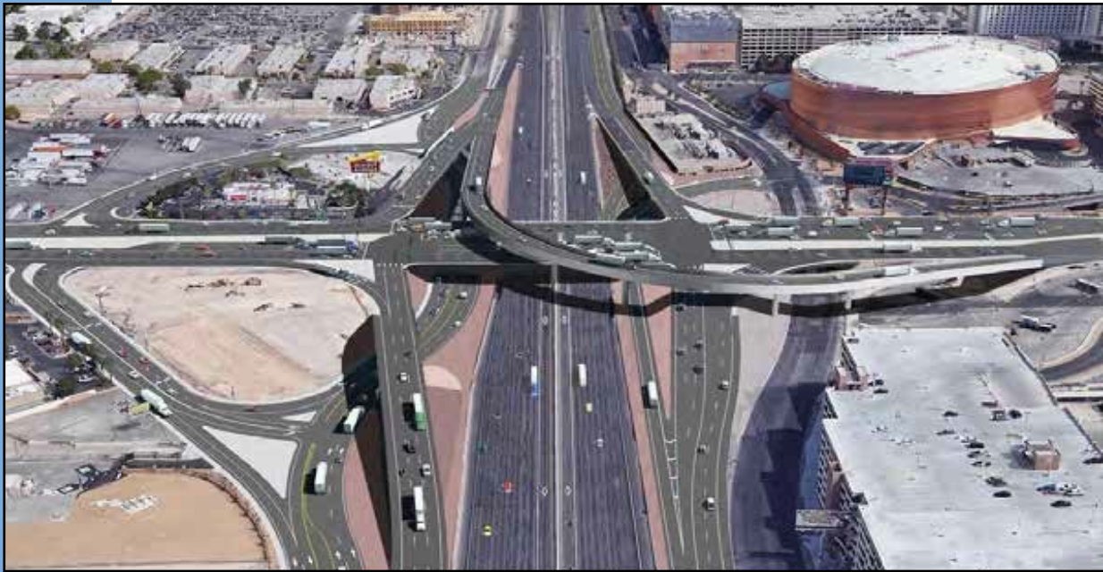
View looking north of the Tropicana Interchange improvements.
