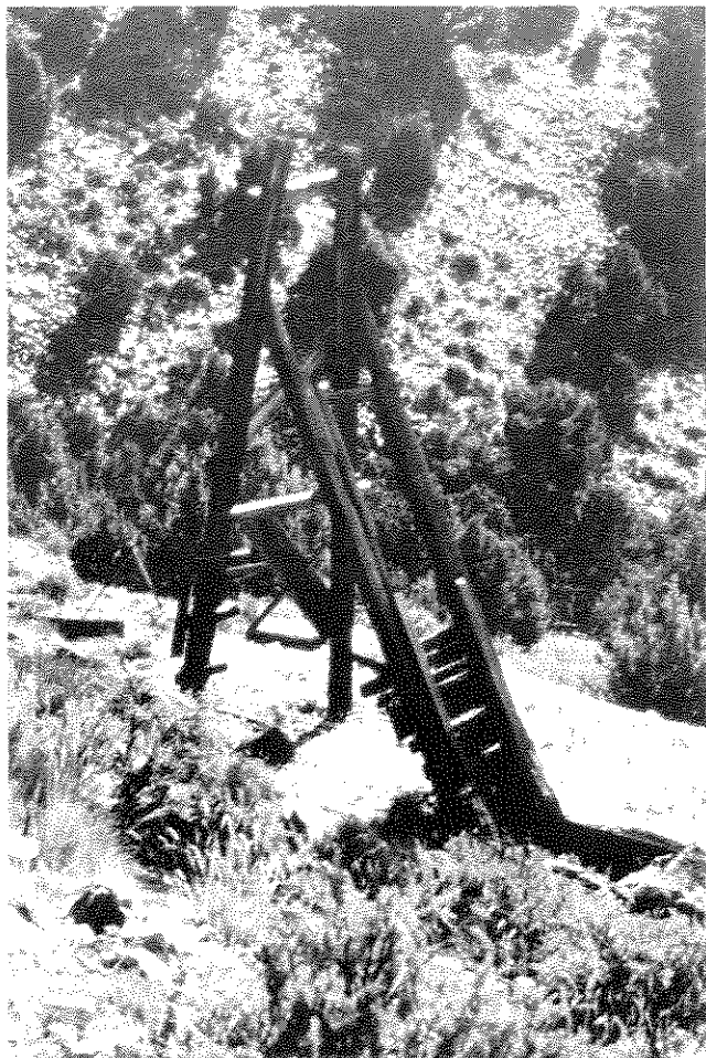
Inclined shaft at the Highgrade mine, Groom district. J. Quade photo.
