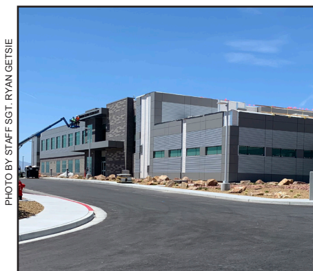
During the biennium, construction completed on the $37 million National Guard Readiness Center. The 70,997 square-foot, LEED Silver certified facility is located on the north end of the Las Vegas Valley, just north of Interstate 15, east of the North Las Vegas Readiness Center, on land already owned by the state.
