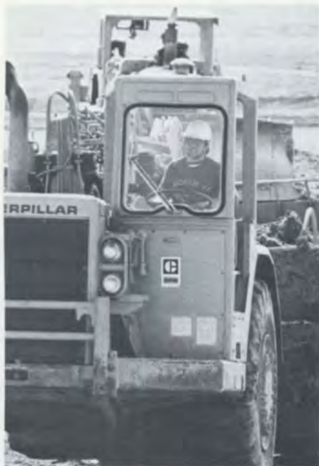
Breaking ground at Freeport mill site.
