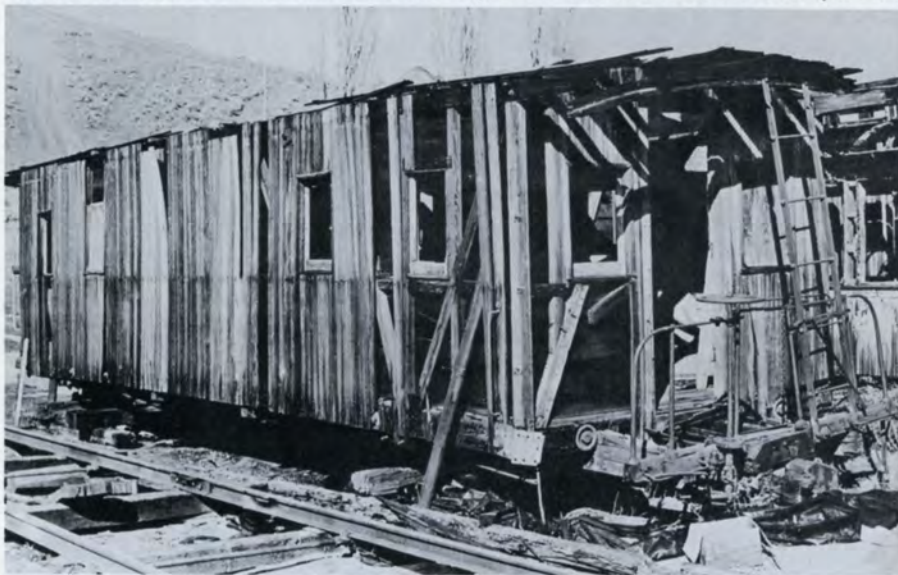
This is what remained of the redwood-sheathed No. 9 caboose before its restoration.
