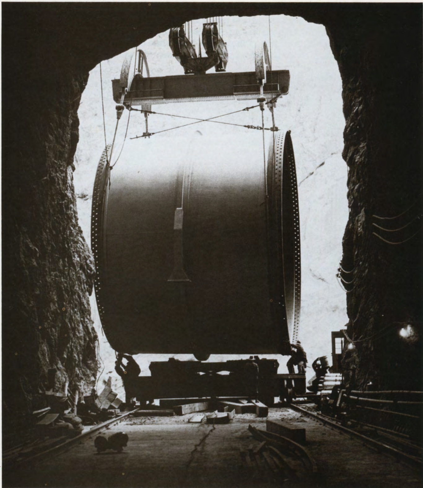
A 30-foot-tall section of pipe weighing more than 150 tons is lowered by cableway into the entrance to a penstock "header" tunnel. The headers received water from the intake towers and directed it to the powerhouse to drive the turbines. Because the pipe sections were too large and heavy to be carried by rail, they were made at a special plant nearby and hauled to the dam by trailer.
