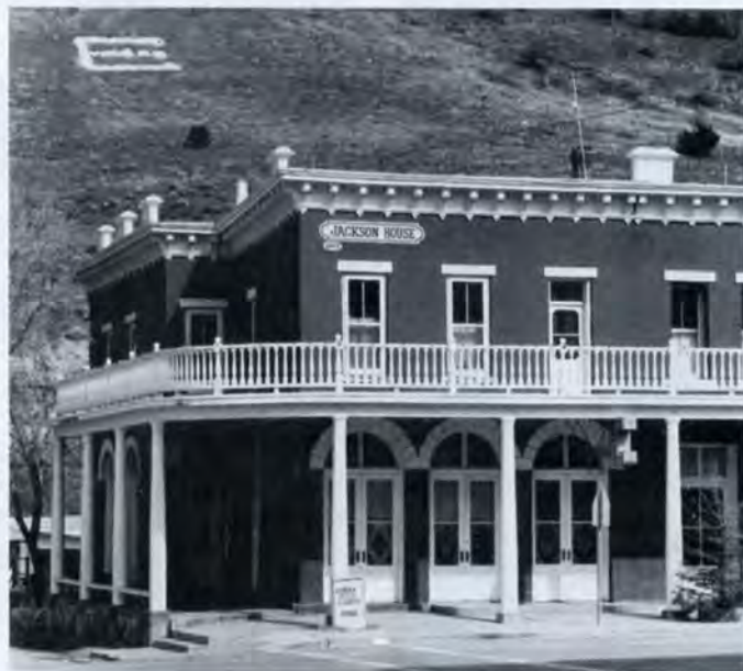
Eureka's Jackson House, an example of rural renewal.
